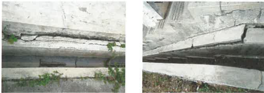
Photo 1.3 Cracked drainage
