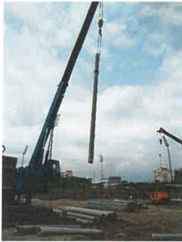
Photo 1.4 : Piling Installation
