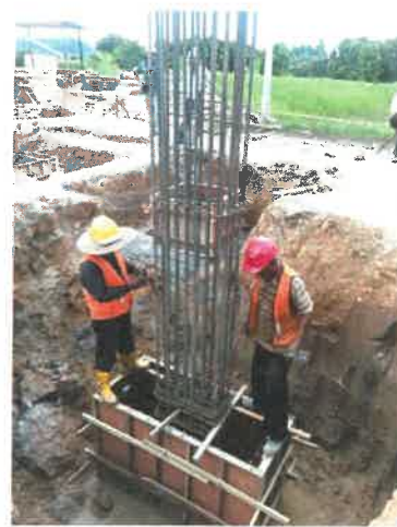
Photo 1.5 : Pilecap and Stumb Installation
