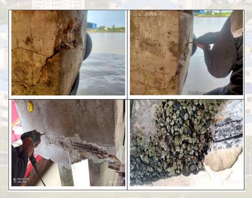
The concrete to be broken out will be marked out by the LMSB. The breakout area shall be entered into record sheet in duplicate and signed by the engineer. The original shall be kept by the Engineer and the duplicate by the LMSB and shall be used as a record for the purpose of measuring the work. Breakout work shall not proceed until approval of the Engineer is obtained.
