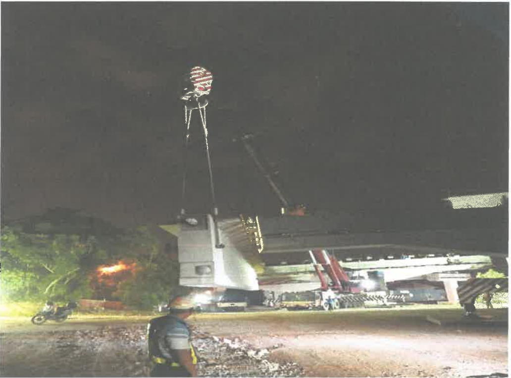
(Launching beam at night)
