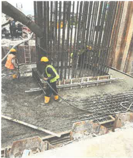
(Process of pouring concrete)
