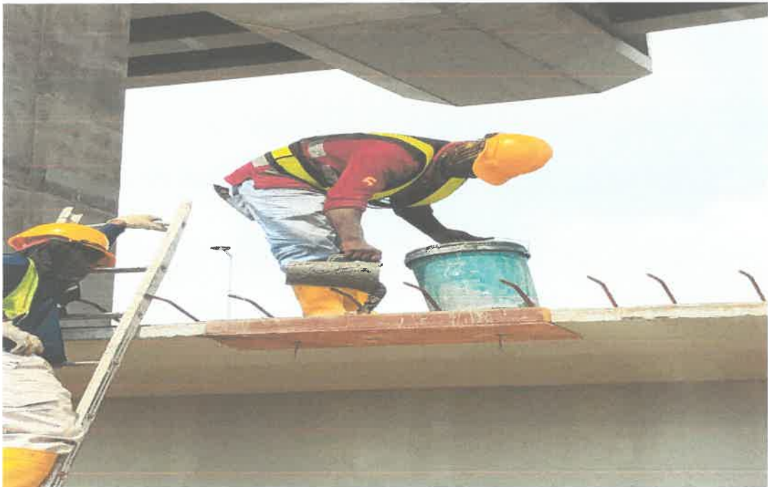
(Fixed the crack of the T-beam)
