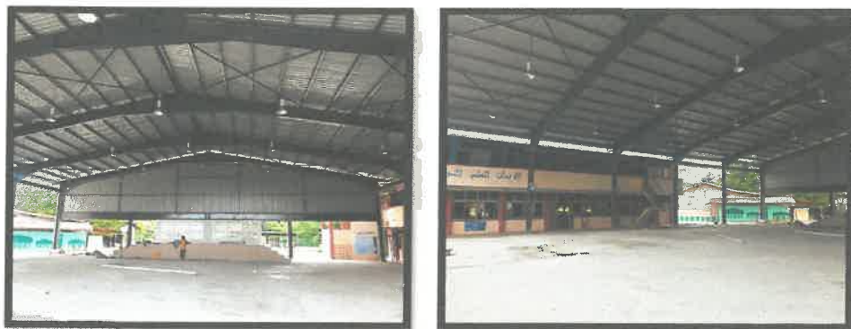
Figure 4.2 : The construction that have been completed.
