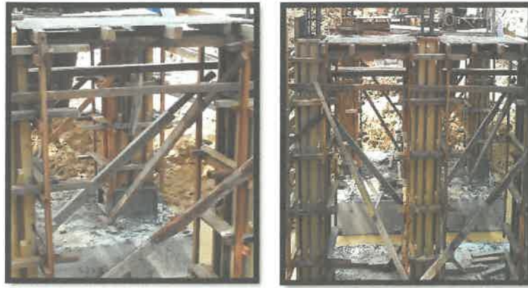
Figure 9.2 : Wood as a material of framework for this project.
