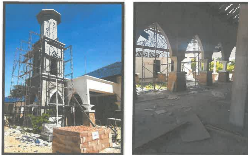
Figure 6 : The process of construction of Masjid Jamek Bahau project.
