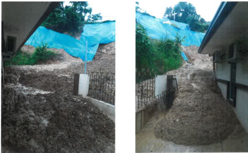
Figure 1.3 Before Site Clearing
