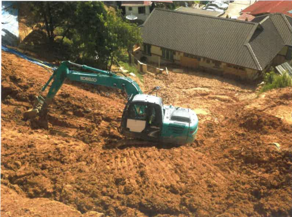
Figure 1.4 During Site Clearing
