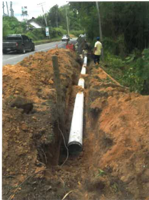
Figure 1.6 Relocation of Drainage
