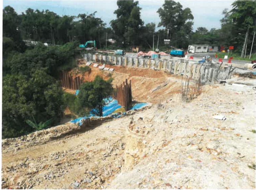
Figure 1.9 Progress photo I
