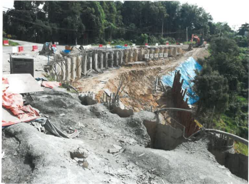
Figure 2.1 Progress photo III
