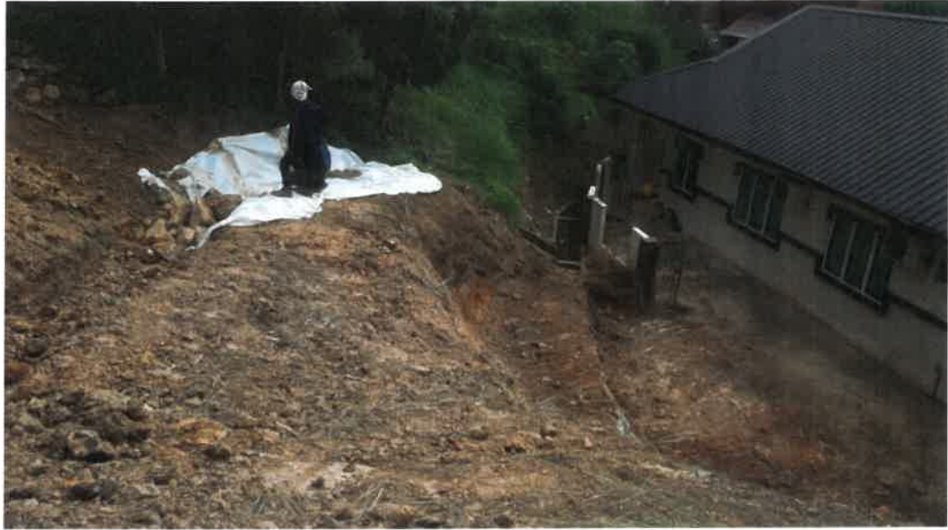
Figure 1.5 After Site Clearing
