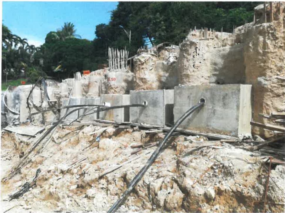
Figure 2.2 Progress photo IV
