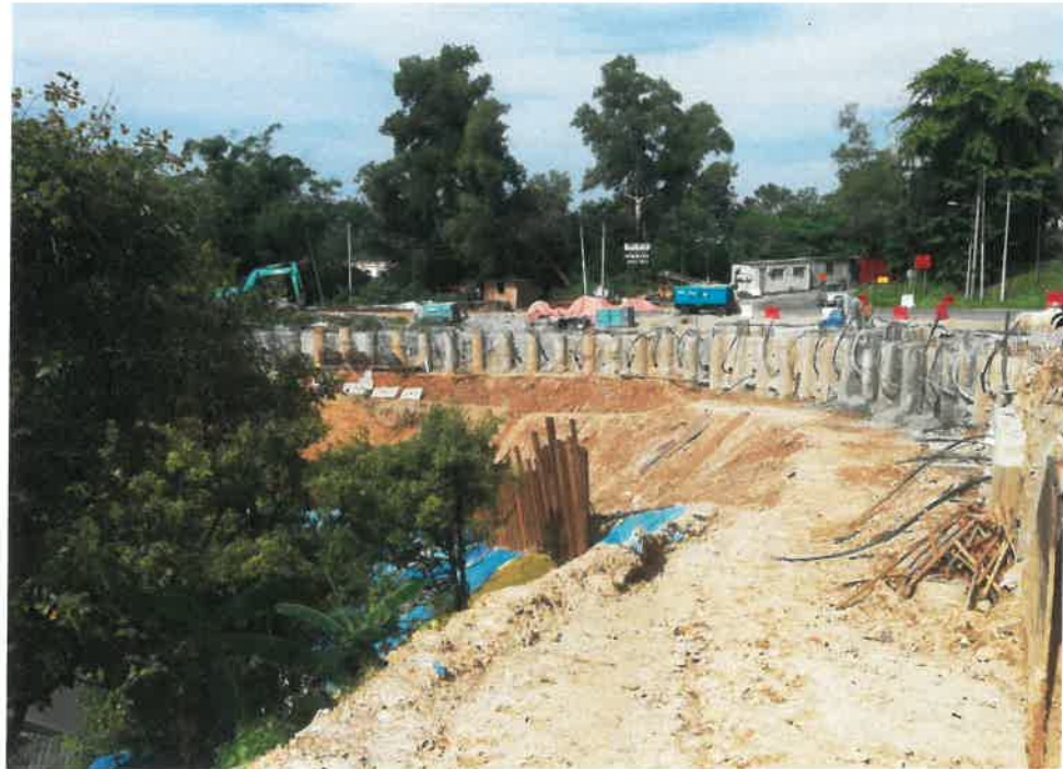
Figure 2.0 Progress photo II
