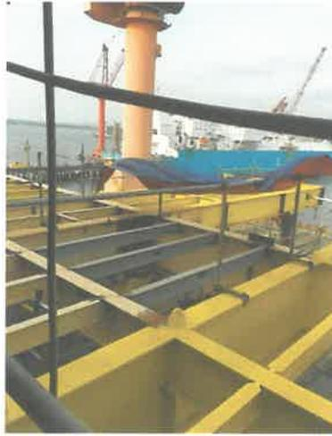
Figure1.3: Example of primary beam attach to secondary beam (I Beam)
