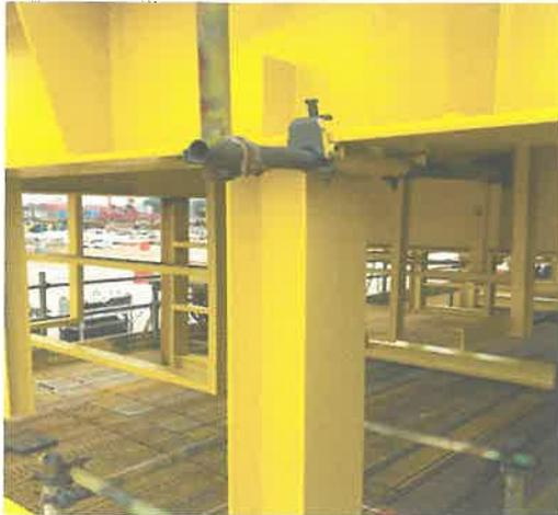
Figure 1.4: Pipe rack after final coat (yellow 550)
