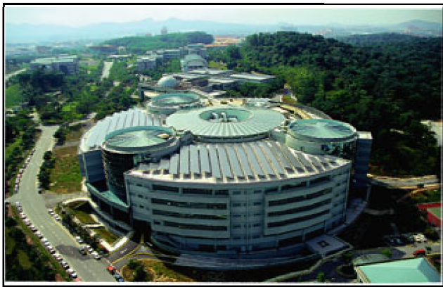
Figure 2. A largest of GCPV system with 361.9 kWp at Enterprise Four Building, Technology Park Malaysia (TPM), Malaysia. (Sources: TPM)
