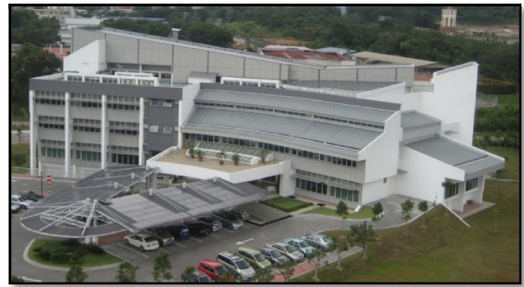
Figure 3. A second largest of GCPV system with 92.00 kWp at Malaysian Green Technology Corporation, Bandar baru Bangi, Malaysia [1].
