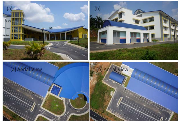
Figure 9: Simulated heritage building (a) Main entrance side view and aerial view (b) Front left side view and aerial view
