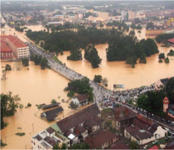
Figure 3 Flood in Bandar Segamat on December 2007 [21]
