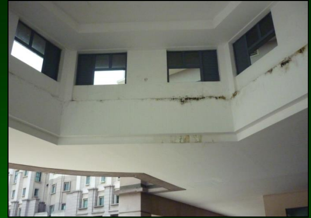
Figure 7.0: The Watermark Cause by Waterproofing Failure at Roof Level at Block 7
