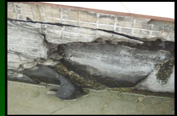
Figure 6.7: The waterproofing already detach from the sub screed
