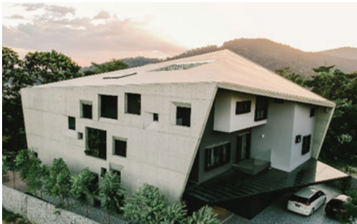
Figure 3. The Windows House, Kuala Lumpur
