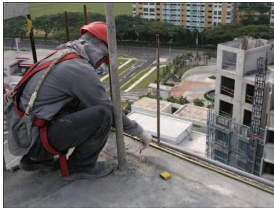
Figure 2.16 : Position And Alignment Checking
