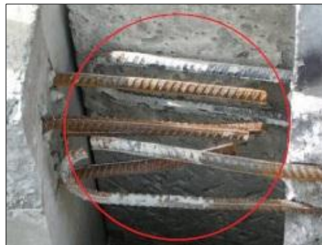
Figure 2.24 : Protruding Bars
