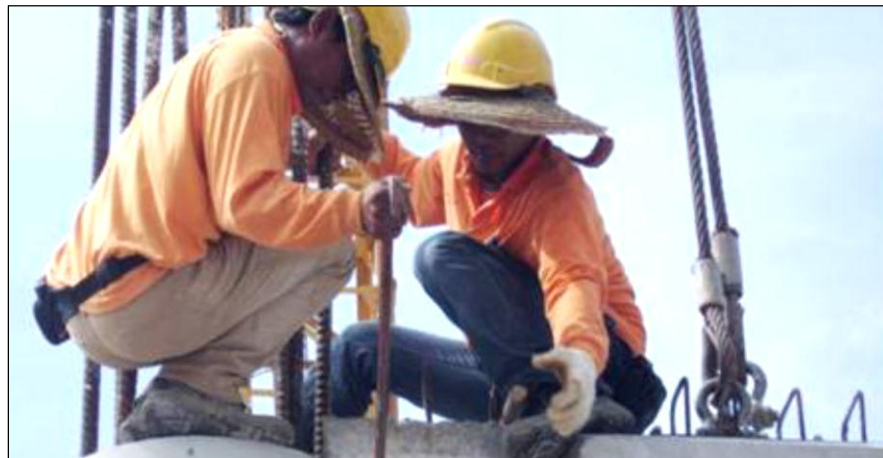
Figure 3.18 : Adjust Beam Proper Seated On Corbel at Site
