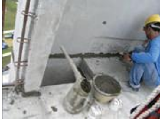
Figure 2.20 : Grouting Process
