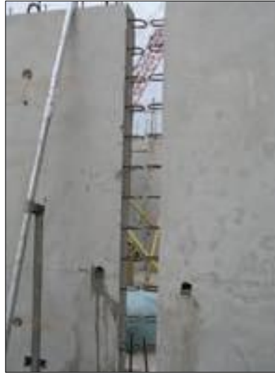
Figure 2.22 : Jointing component process
