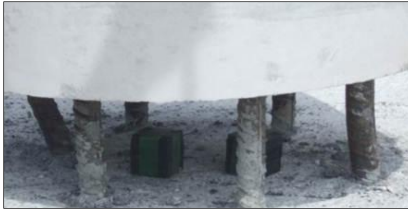
Figure 3.13 : Column Seated On The Top Shim Plate at site
