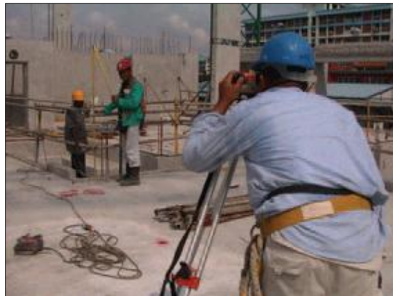
Figure 2.14 : Alignment Checking
