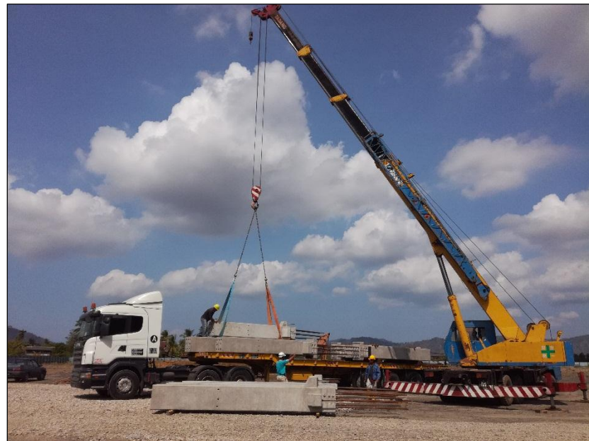
Figure 3.9: Component Precast Column And Beam Arrived At Site
