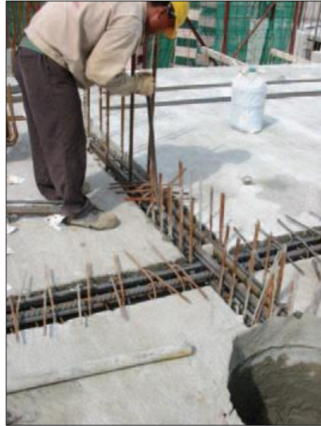
Figure 2.28 : Jointing Process
