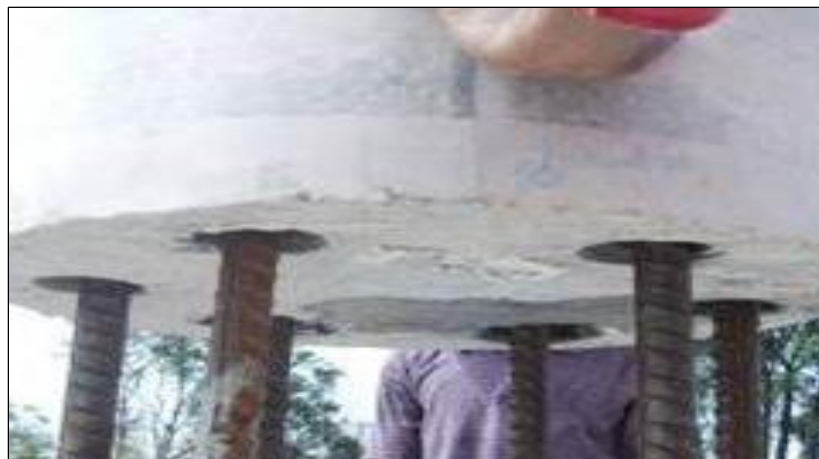
Figure 3.15 : Column Starter Bar Slot Into Duct At Site
