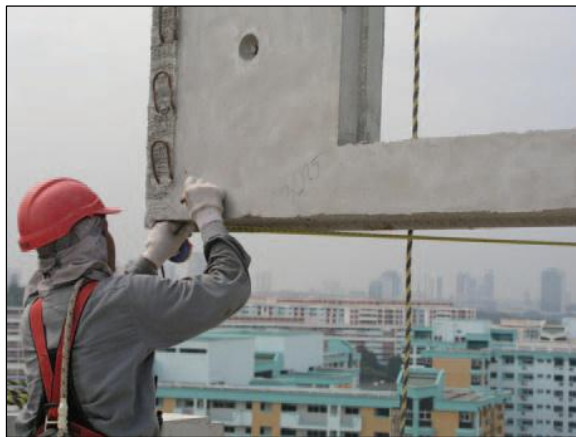
Figure 2.17 : Backer Rod Checking
