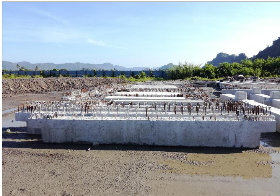
Figure 3.4 : Beam Component At Site
