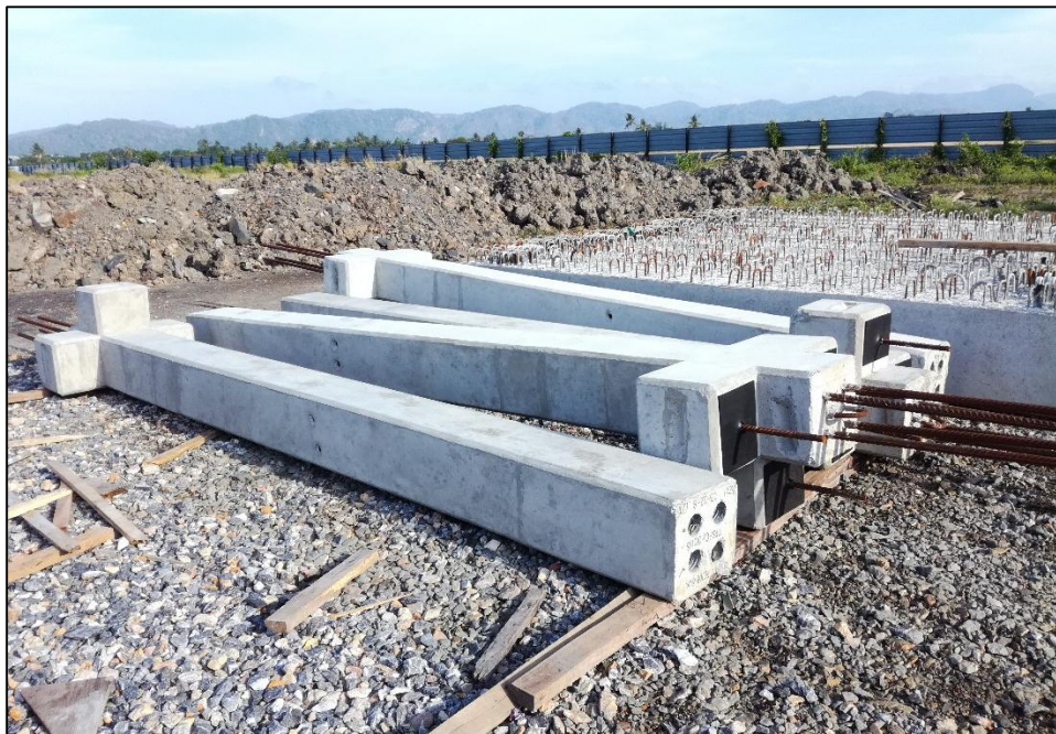
Figure 3.3 : Column Component At Site
