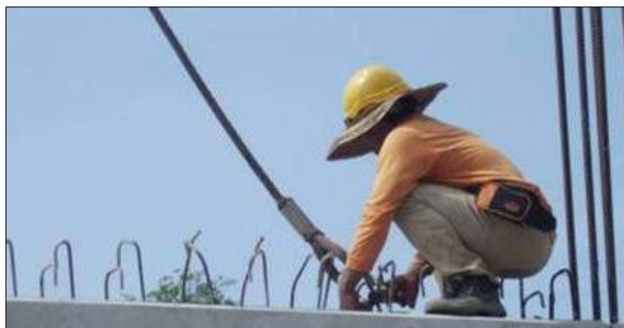
Figure 3.19 : Remove of Shackle, Wire Rope
