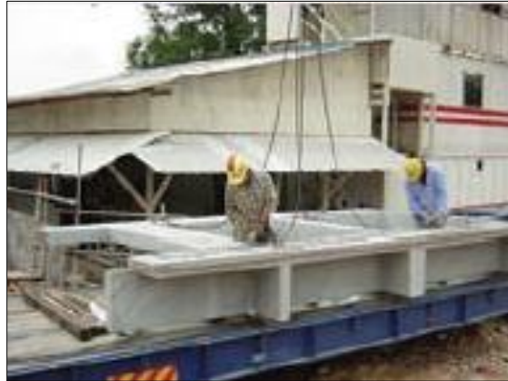
Figure 2.12 : Inspection On Concrete
