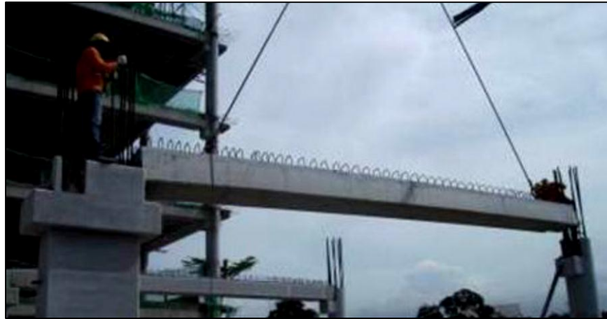
Figure 3.17 : Beam Slot Into Dowel Bar at Site
