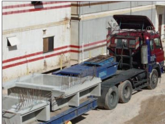
Figure 2.10 : Delivery Of Precast Component
