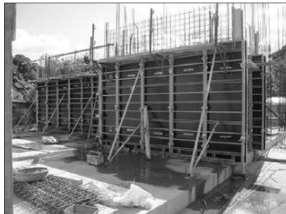
Figure 2.2 : Steel Formwork System
