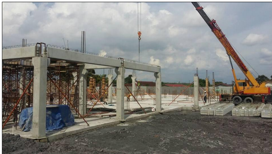
Figure 3.16 : Installation of Precast Beam at Site
