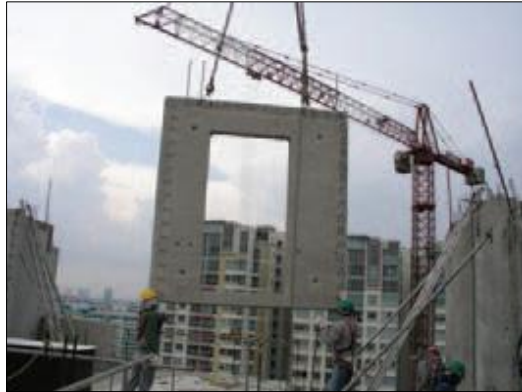
Figure 2.18 : Precast Component Lifting
