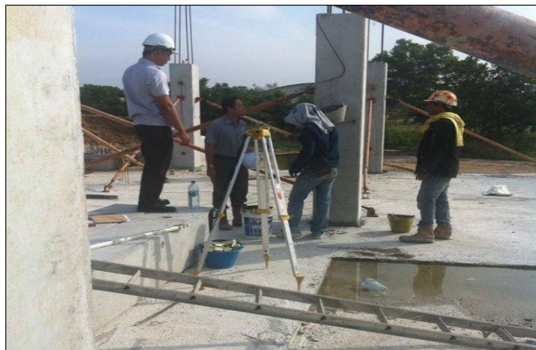
Figure 3.12 : Vertically, Alignment of Precast Column At Site
