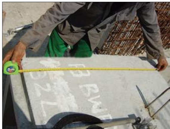
Figure 2.11 : Measurement Check For Precast Component
