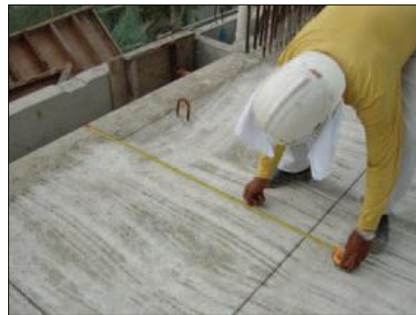
Figure 2.23 : Setting Out Process
