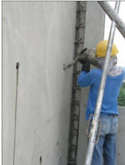
Figure 2.21 : Grouting Process
