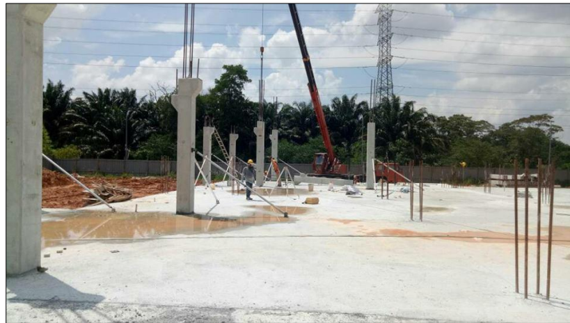
Figure 3.14 : Installation of Pull Push Props At Site
