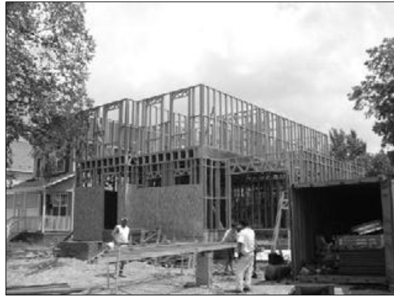
Figure 2.3 : Steel Framing System
