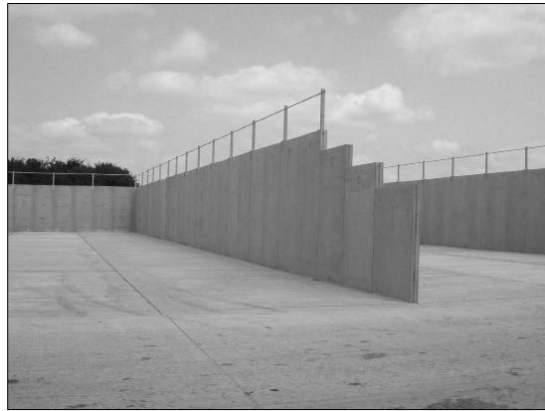
Figure 2.1 : Precast Concrete Wall
