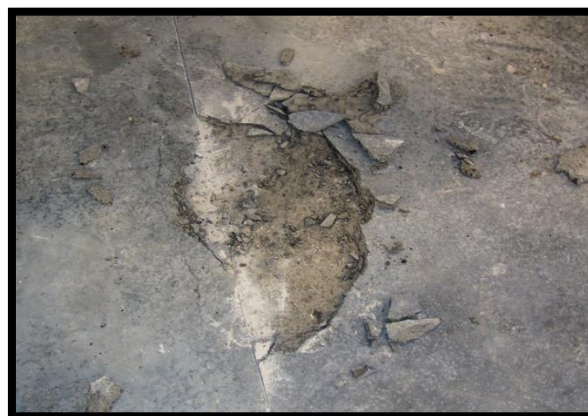
Figure 2.16: the slab surface contain blister
