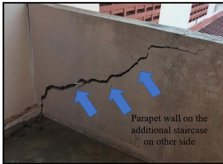
Figure 3.10: the view of parapet on other side
