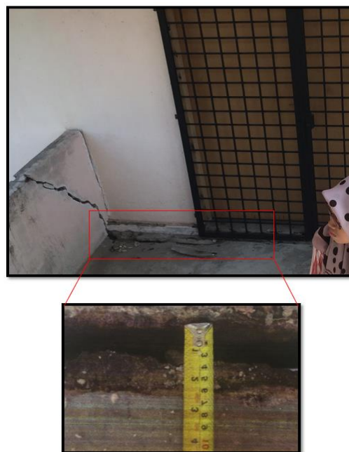
Figure 3.22: strain on staircase slab.
