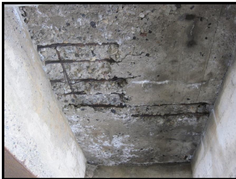
Figure 2.14: the example of concrete spalling by corrosion
