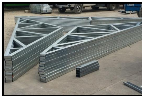
Photo 24 – Cold-Formed Steel Trusses
