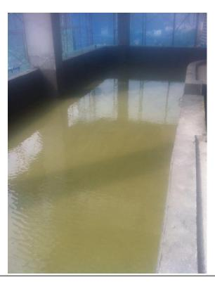
WATER PROOFING FOR PONDING TEST AT SWIMMING POOL LEVEL 14
