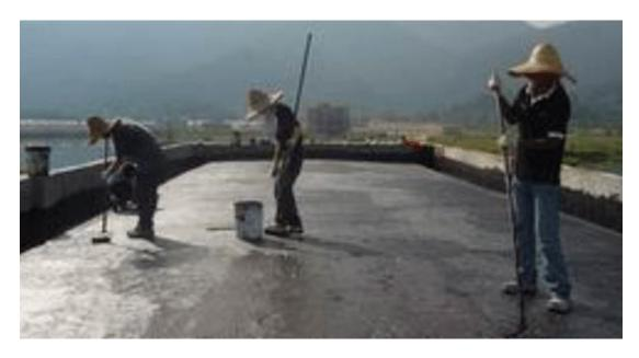
Figure 2.12 Bituminous coating waterproofing
