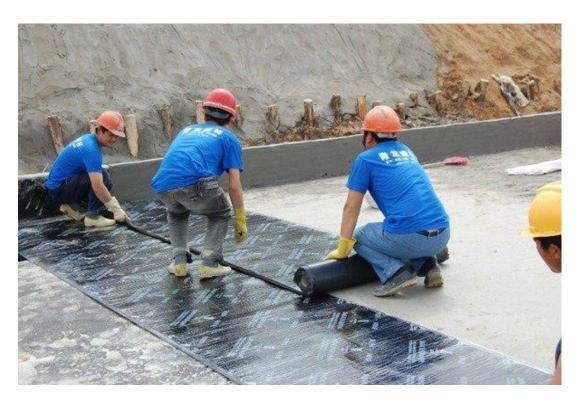
Figure 2.13 Bituminous membrane waterproofing
