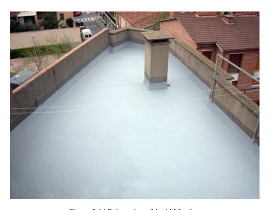
Figure 2.14 Polyurethane Liquid Membrane
