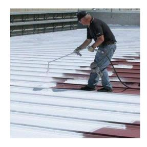
Figure 2.11 Liquid waterproofing membrane
