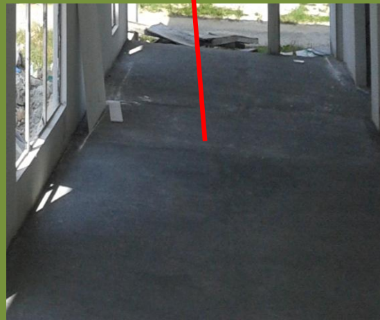
Figure 3.12 The Concrete Floor
