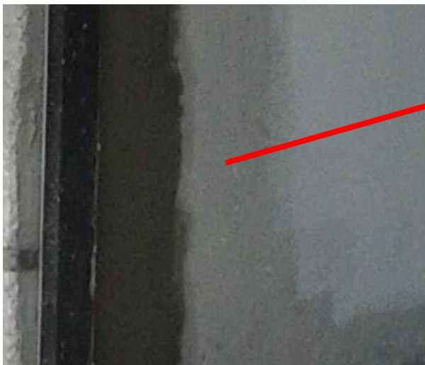
Figure 3.7 The Layer Of Plastering
