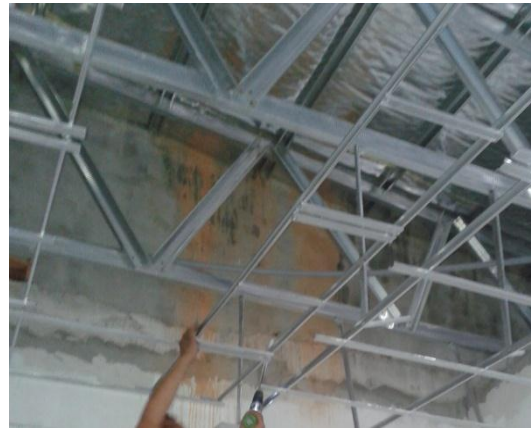
Figure 3.27 The Process Of Ceiling Framework Installation
