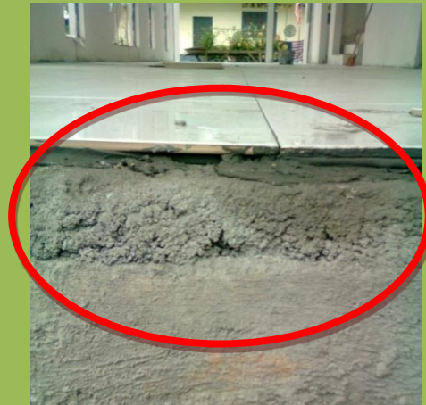
Figure 3.22 The Layer Of Floor
