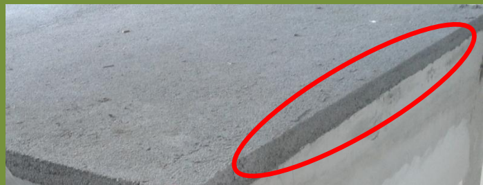
Figure 3.13 The Layer Of Cement Mixture Before Ceramic Installation
