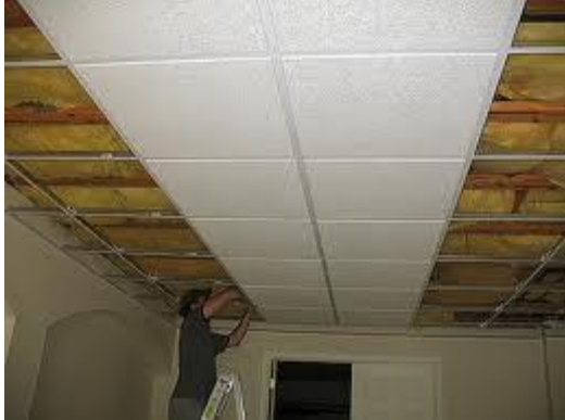
Figure 2.8 The Suspended Ceiling
