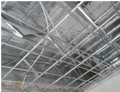
Figure 3.28 The Framework Has Be Complete.
