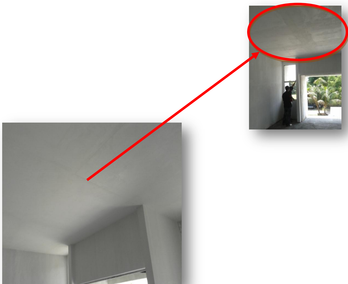
Figure 3.11 The Lime Stone Ceiling
