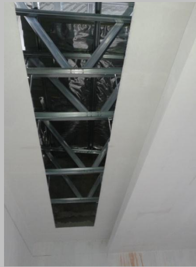
Figure 3.29 The Ceiling Was Be Install
