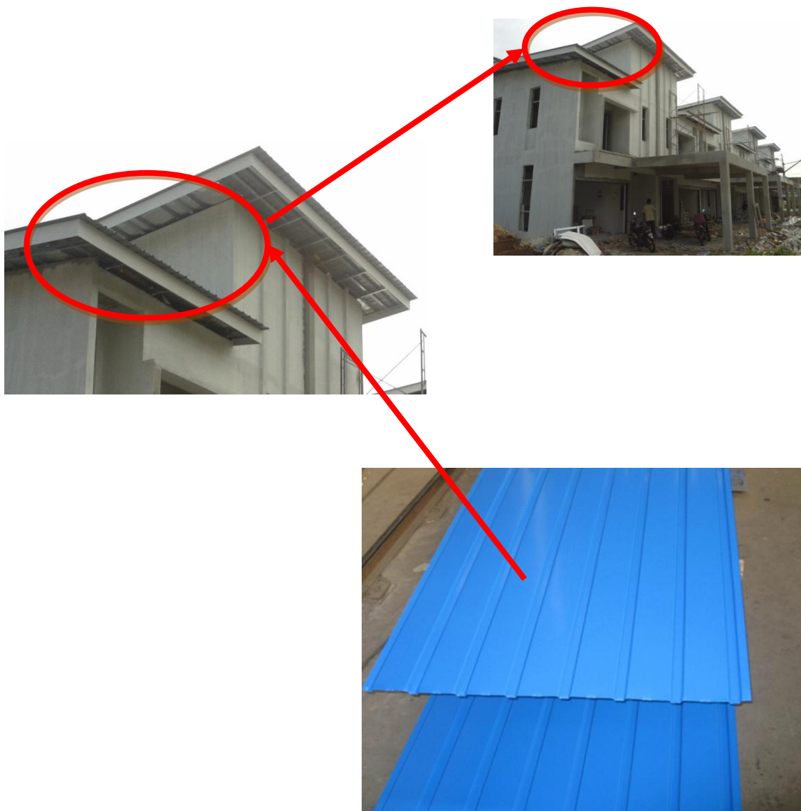
Figure3.9 The Type of Roof Metal Deck
