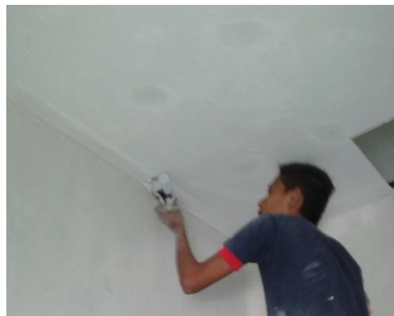
Figure 3.30 The Process Sweep By Using Plaster White Cement.
