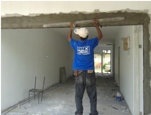
Figure 3.6 The Plastering Process
