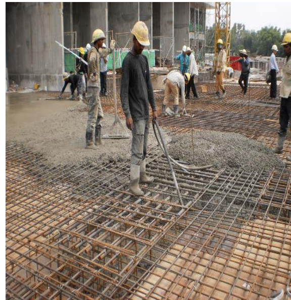
Photos 3.106 : Compacting of concrete using by vibrator
