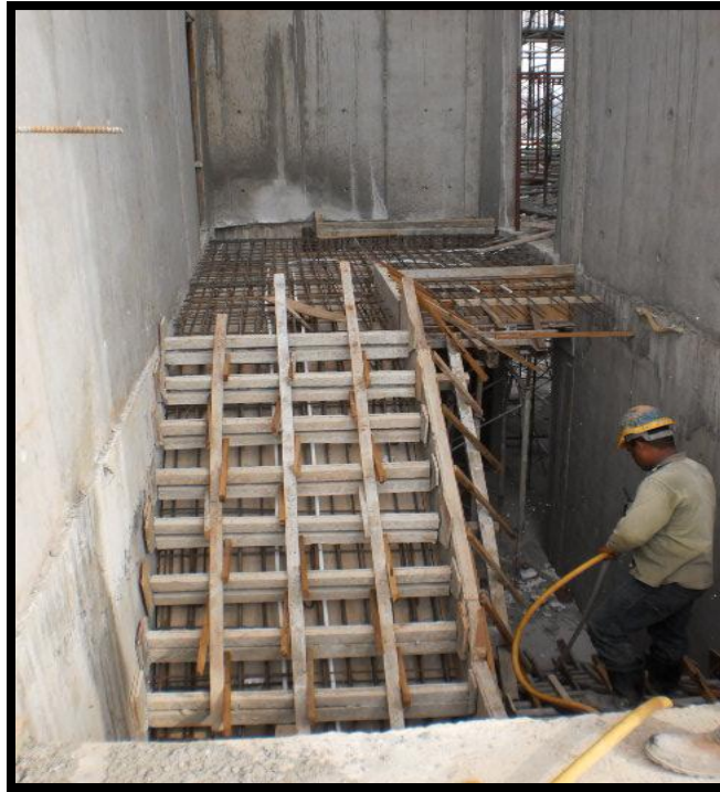
Photos 3.110 : Before concreting work for staircase
