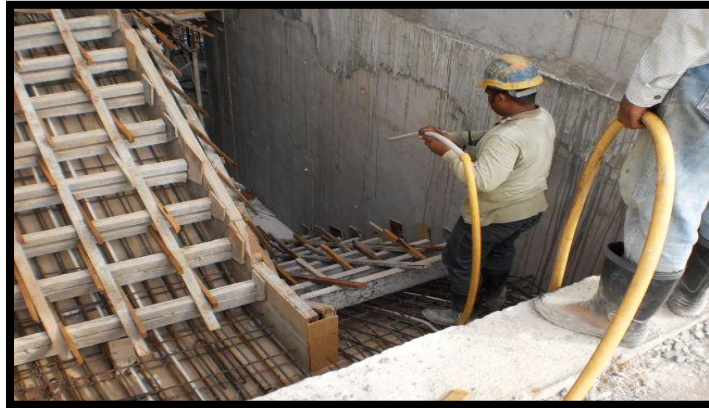
Photos 3.13 : The example of cleaning work using the blower pipe.
