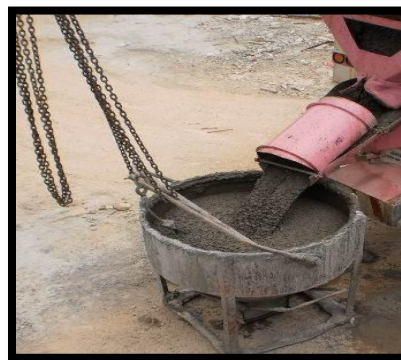
Photos 3.36 : Concrete ready mix from batching plant
