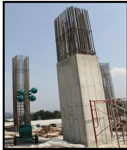
Photos 3.109 : After the concreting work (1 st Cast) for Large Column Hotel
