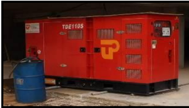
Photos 3.11 : Generator used to generates tower crane at Hotel Apartment.
