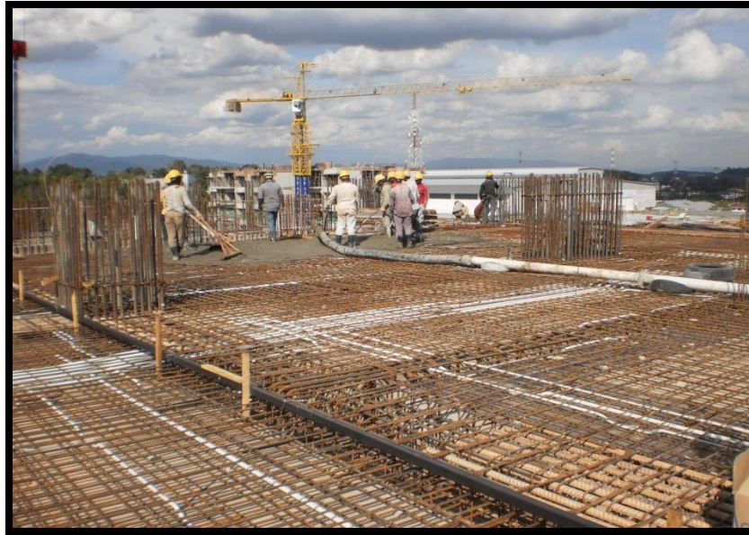
Photos 3.102 : Concreting work for slab at Hotel Aras 5
