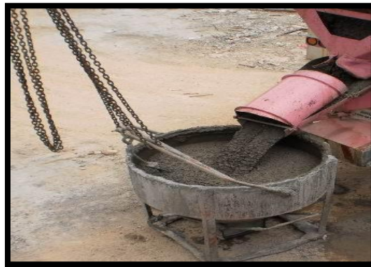
Photos 3.18 : Standard Concrete Bucket for 3m cubes
