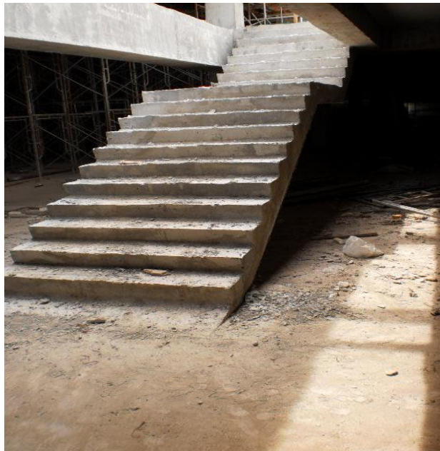
Photos 3.111 : After all concrete work for staircase has been completed
