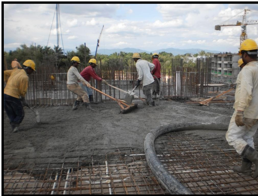
Photos 3.103 : Concreting leveling work
