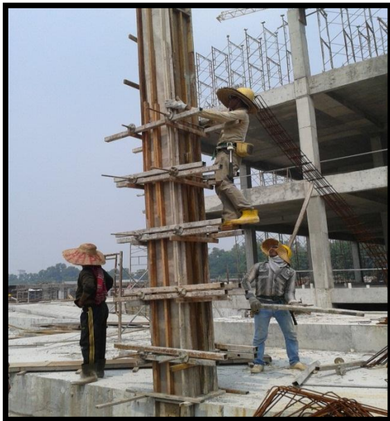
Photos 3.108 : Installation of formwork for Small Column
