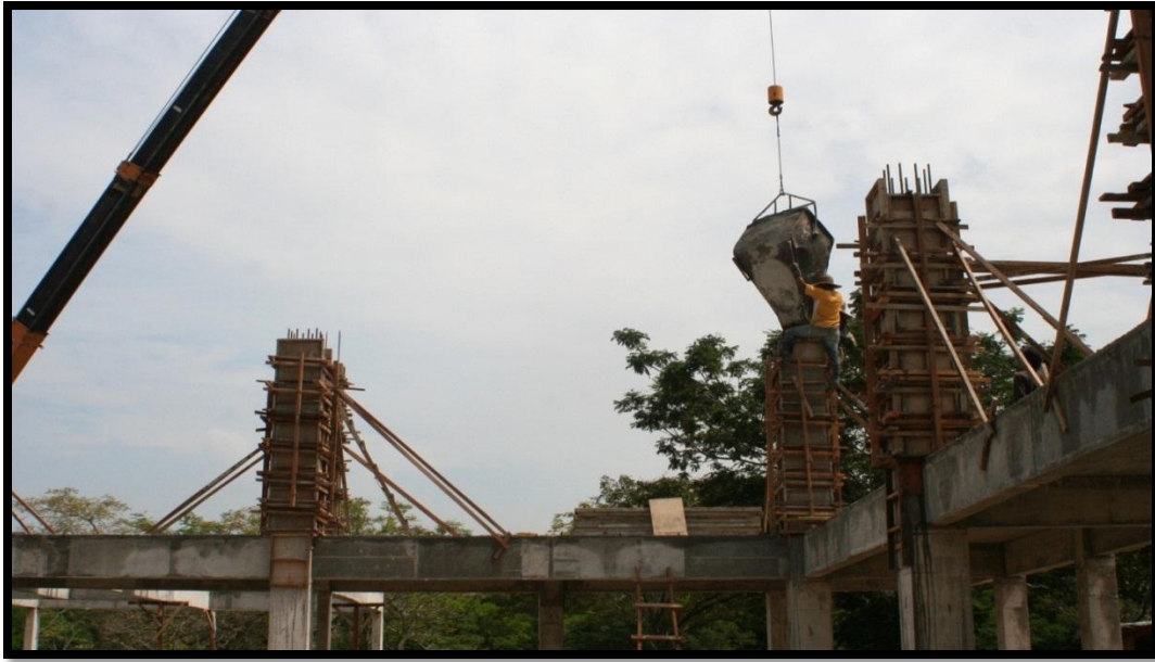
Photos 3.107 : Concreting work for Large Column
