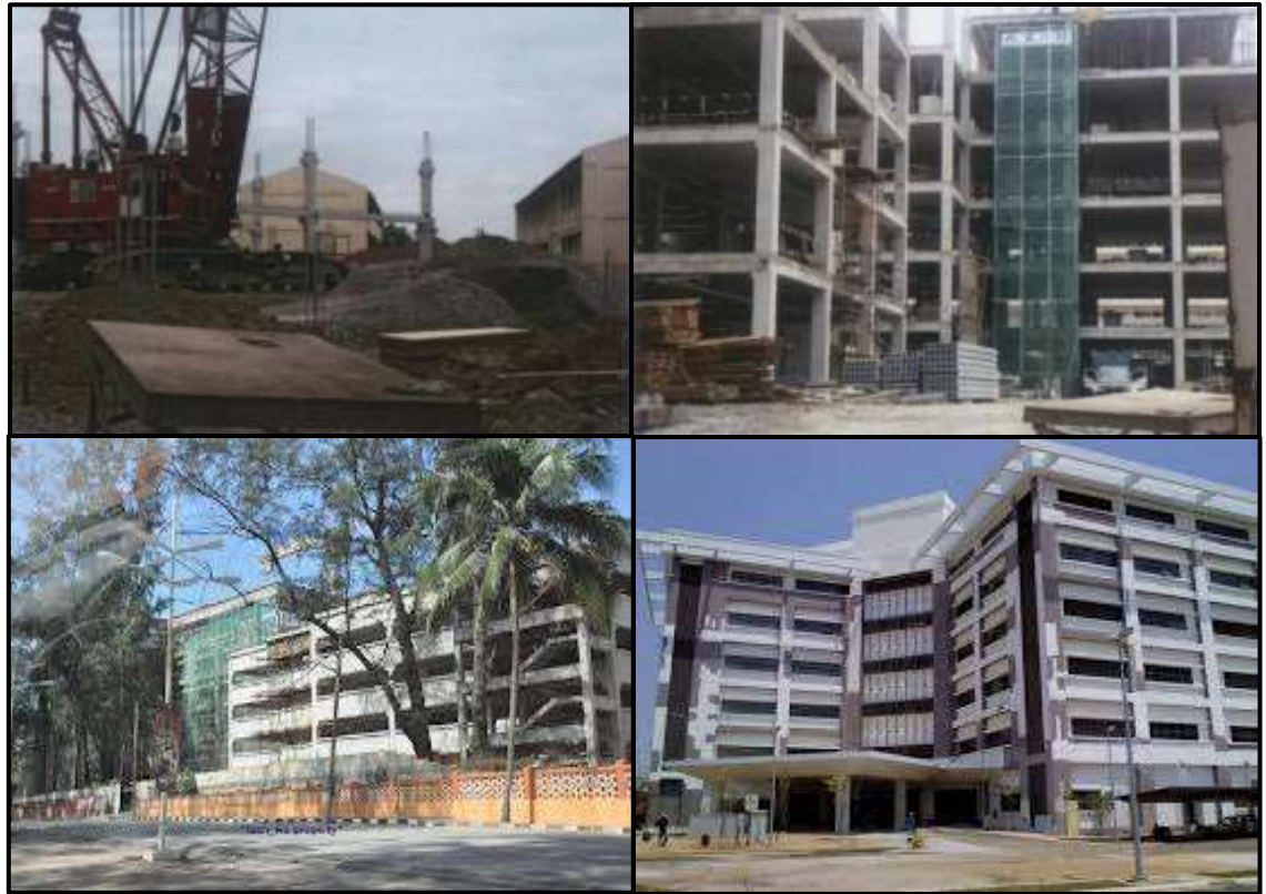
Photo 3.11 Construction Process From One Stage To Next Stage
