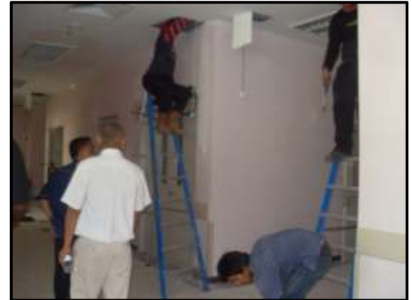
Photo 3.13 Workers Do Electrical Works
