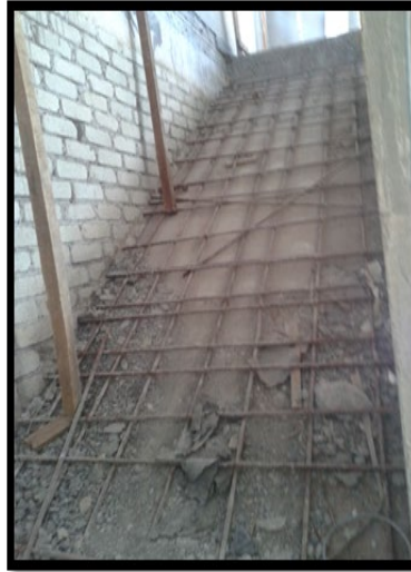
Figure 3.3.1.5: Installation Of reinforcement steel
