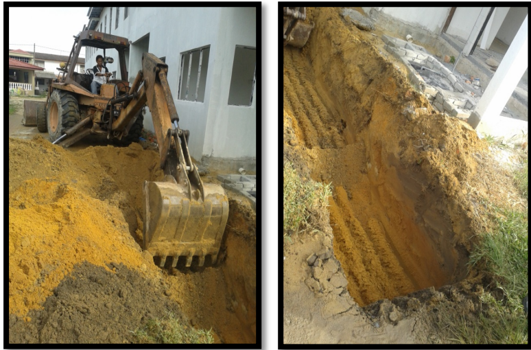
Figure 3.2.1.2: Excavation Work Done
