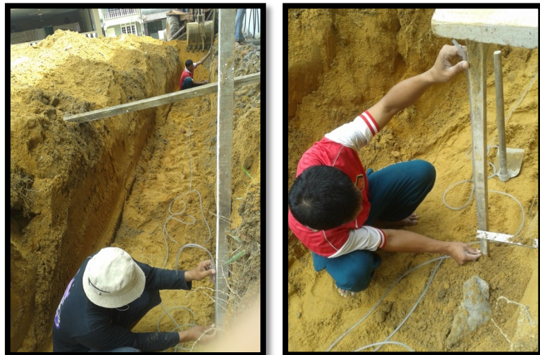
Figure 3.2.1.5: Levelling Process
