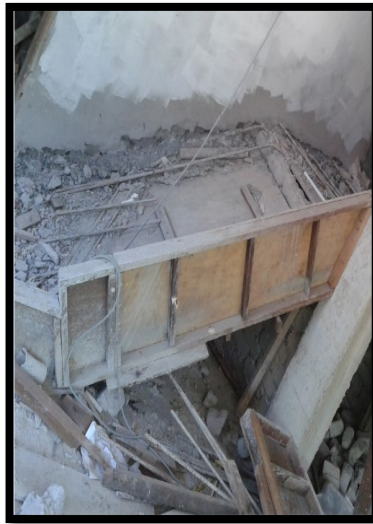
Figure 3.3.1.1: Formwork of Staircase
