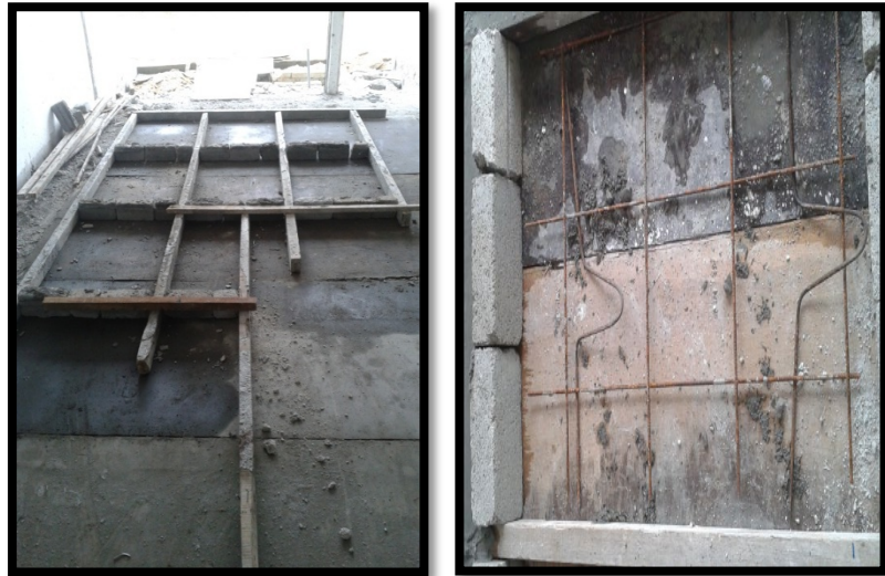
Figure 3.2.2.2: Formwork of Drain Figure 3.2.2.3: Hold of Drain Cover
