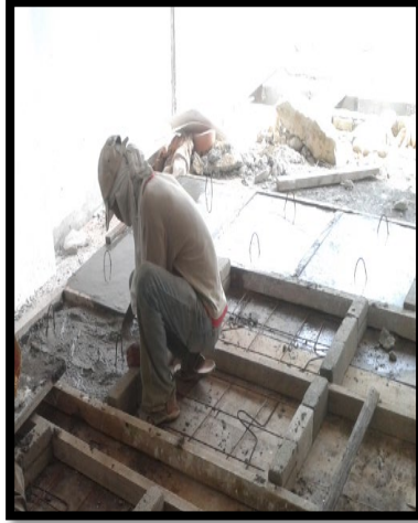
Figure 3.2.2.4: Poured Concrete Mixture into Formwork
