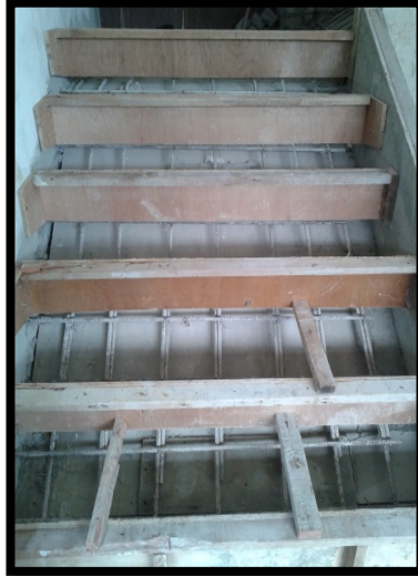
Figure 3.3.1.6: Formwork for Thread and Riser.
