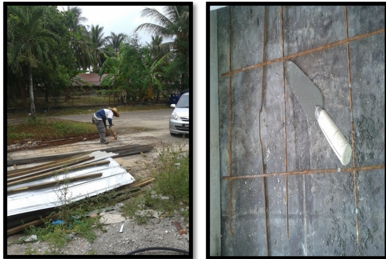
Figure 3.2.2.1: Cutting the Bar Reinforcements Concrete (Brc)
