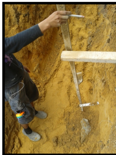
Figure 3.2.1.3: Pouting the Timber in Soil
