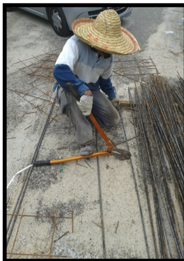
Figure 3.3.1.3: Cutting the Reinforcement Steel Y12
