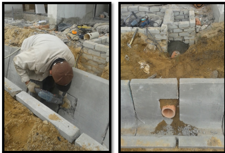
Figure 3.2.1.7: Drill of Drain
