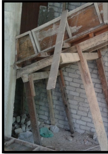
Figure 3.3.1.2: Timber as a Retainer
