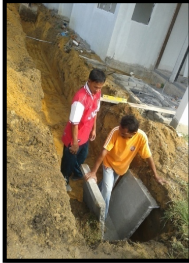
Figure 3.2.1.6: Installation of Drain
