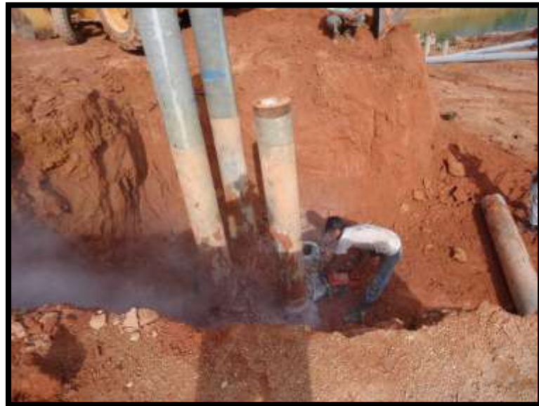
Figure 3.5.13 Cut of Piles
