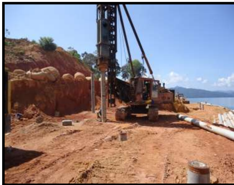
Figure 3.5.7 Piles Lifting the Hammer
