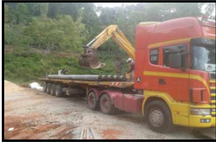
Figure 3.5.4 Supply and delivery pile
