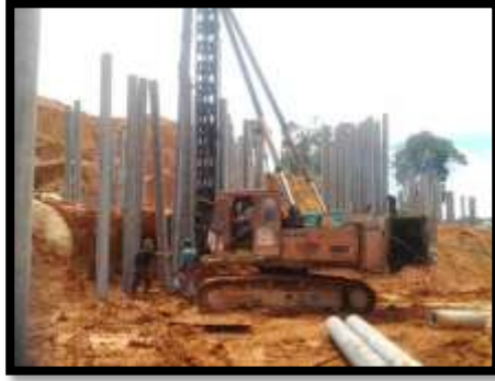
Figure 3.7.7 Hydraulic Piling Hammer
