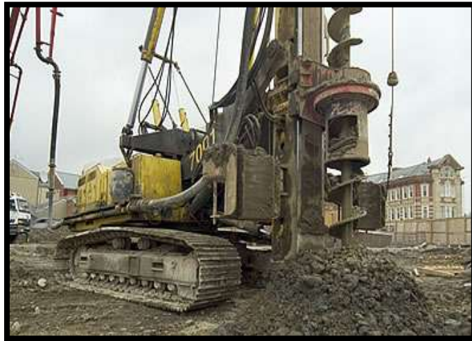
Figure 2.4.2: Continuous Flight Auger
