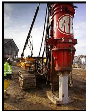
Figure 2.4.1: Pre-Cast Concrete Piles
