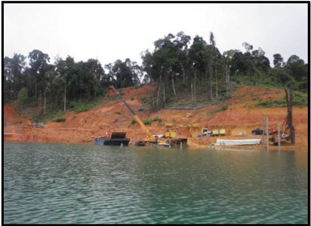
Figure 3.2.1: View of the piling work on the lake edge.
