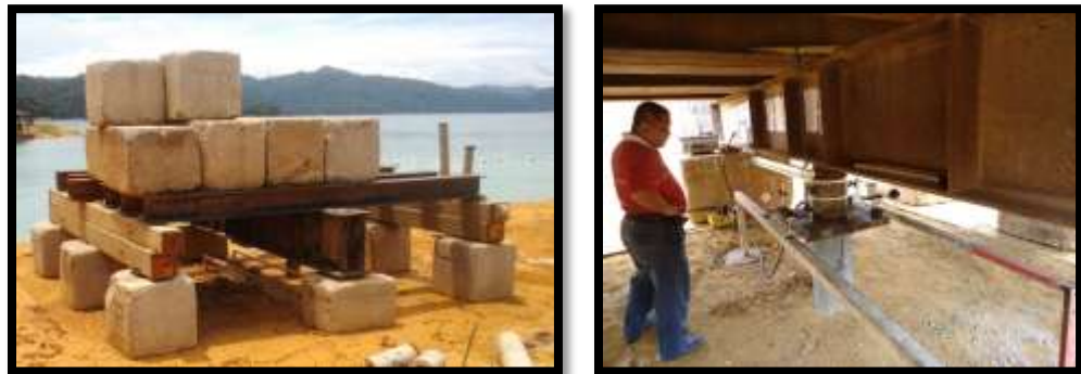
Figure 3.6.1 Load Test for Site
