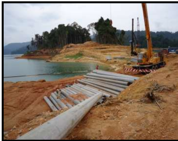
Figure 3.5.5 Cranes and Place the Piles
