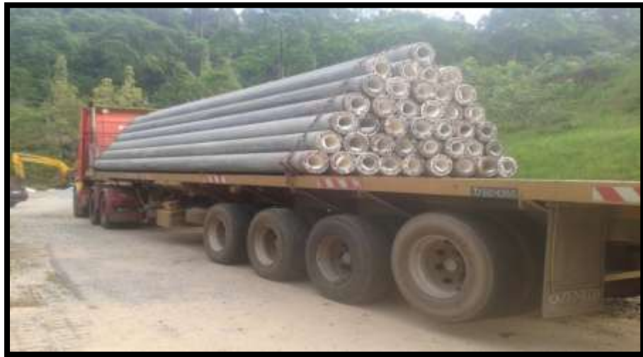
Figure 3.3.2 Delivery Pile to Site
