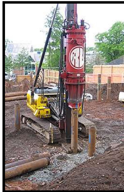
Figure 2.4.3: Tubular Steel Piles Unrestricted Access
