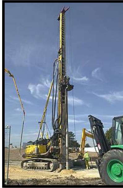
Figure 2.4.4: Bored Displacement Piles
