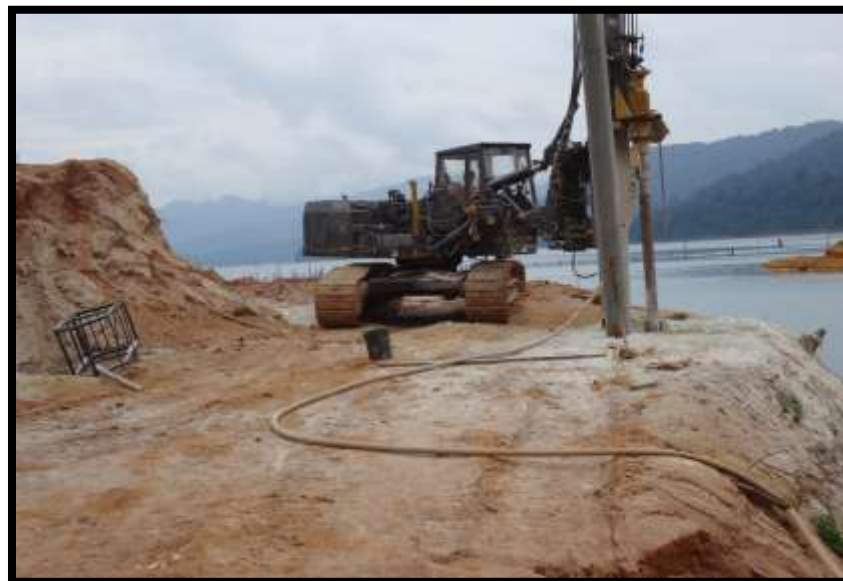
Figure 3.5.9 Lift the Extension Pile
