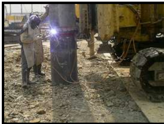
Figure 3.5.11 Welding for Extension Piles
