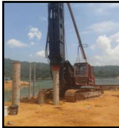
Figure 3.5.3 Hydraulic Piling Hammer
