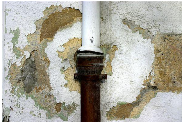
Figure 1.7 Stain on wall surface
