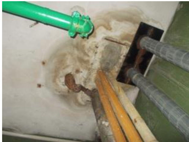
Figure 2.1 Water mark on ceiling
