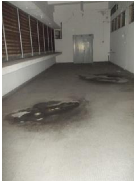
Figure 1.9 Water mark on the floor
