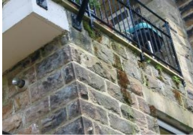
Figure 1.5 Dampness due to rain water
