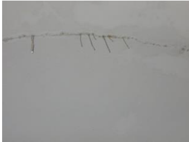
Figure 2.2 Water mark on ceiling surface
