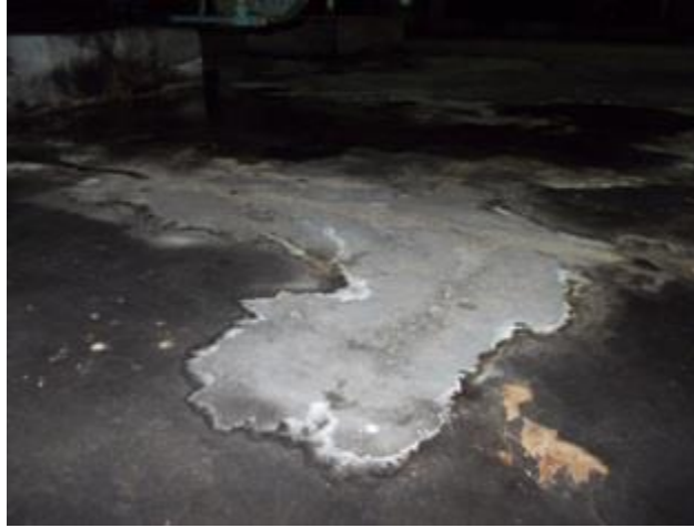
Figure 2.0 Water mark on the floor
