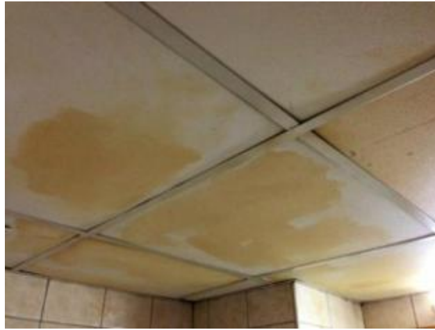
Figure 1.6 Stain on ceiling
