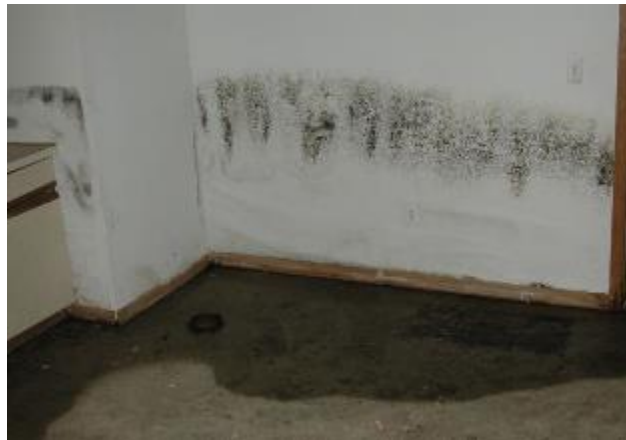
Figure 1.4 Dampness due to ground water
