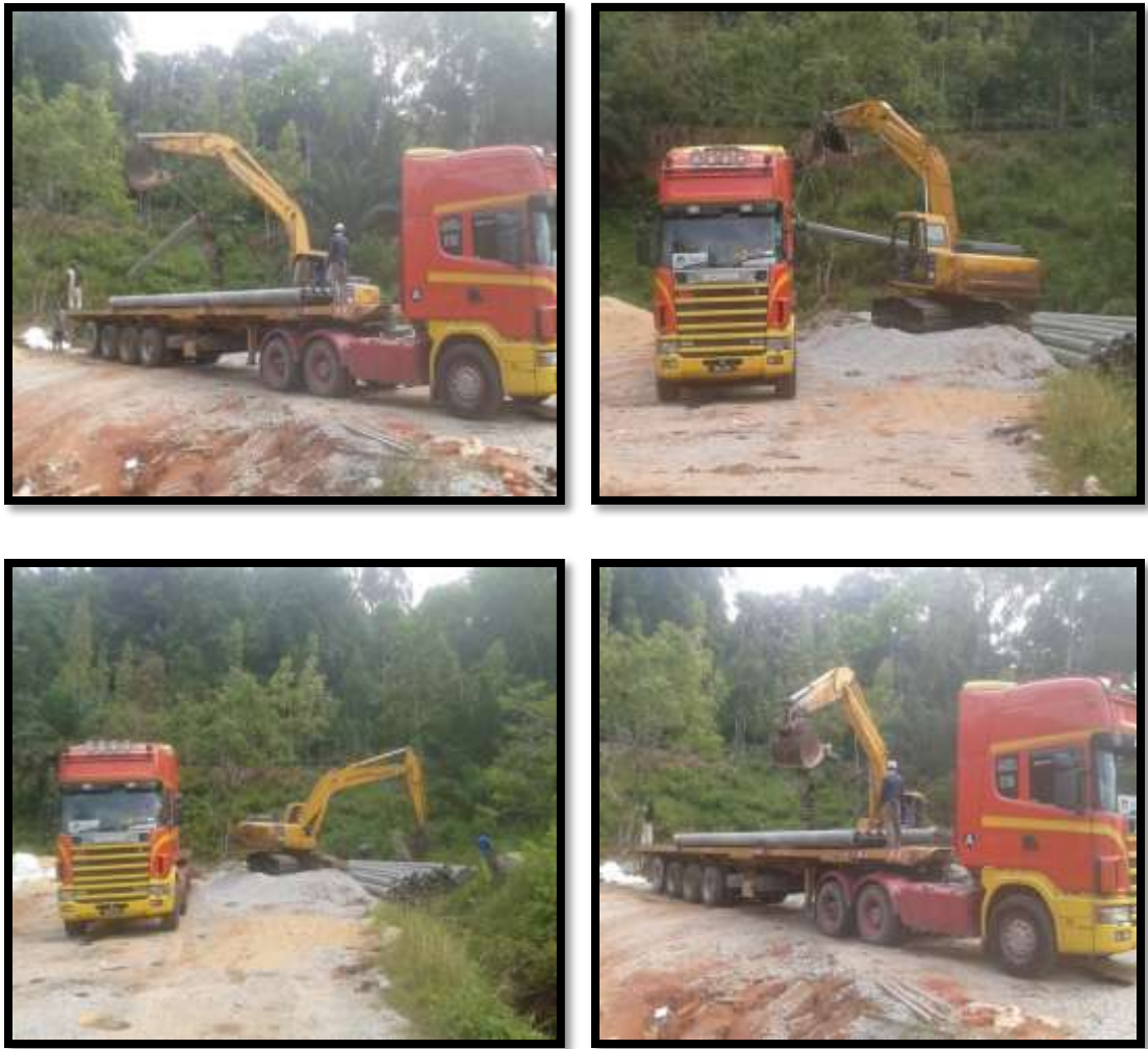
Figure 3.5 shows the transfer piling works on the ground
