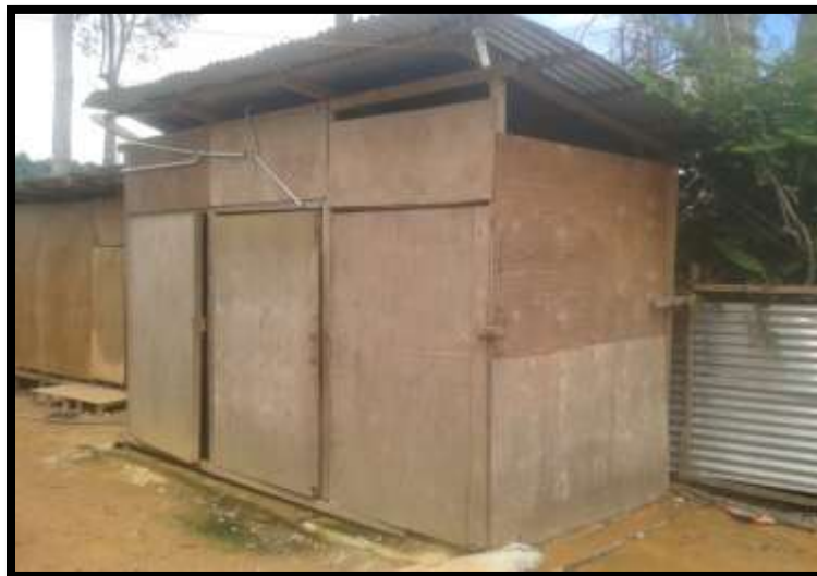
Figure 3.18 show the bathroom and toilet
