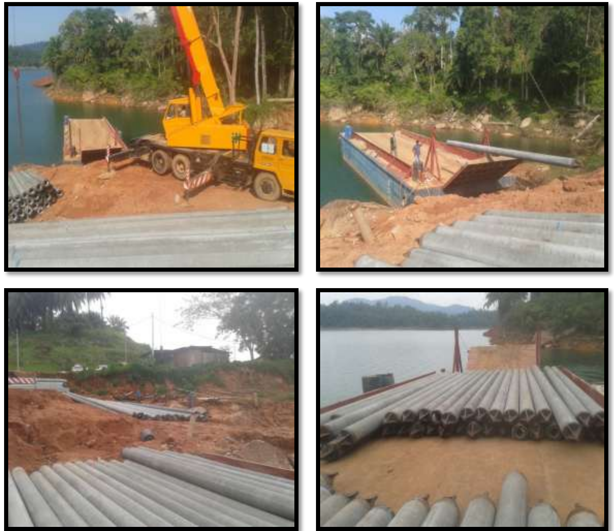
Figure 3.6 shows the transfer piling work into ‘ kapal tokang’
