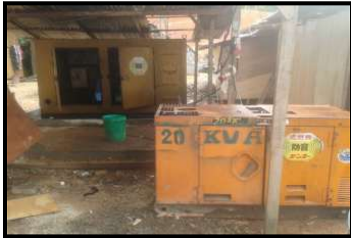
Figure 3.20 show the Generator Set.
