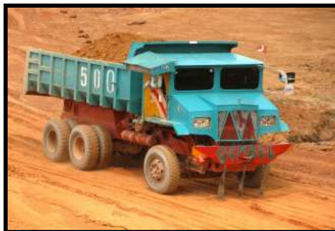
Figure 2.2 : Examples of Machinery at site
