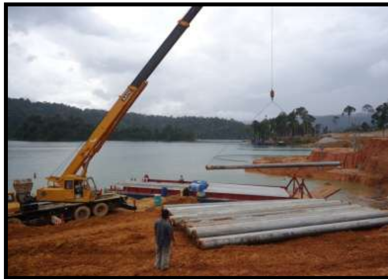
Figure 3.8 shows the works moving pile on site
