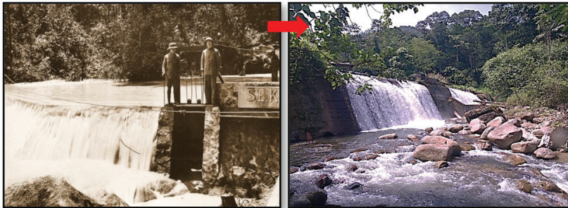
Photo 12: Ulu Geroh dam, built in early 1900s as main water source for tin mining production in Gopeng. Source: Old image courtesy image by Tan Sri Hew See Tong (Left image); Image on the right-photograph by author in 2013.
