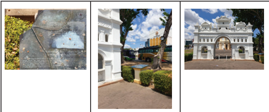
Figure 6. Pedestal Interpretive Sign at Archway Replica of Istana Kota Tengah. The glass top of the Panel is Partly Broken and very Unsightly
