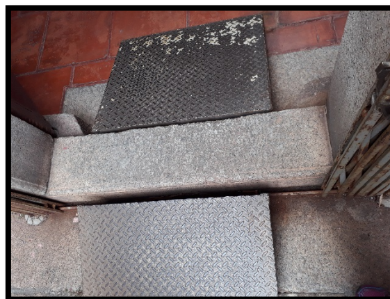
Photo 4: The initiative ramp to provide facilities passage for the Senior citizen and disabilities.
