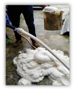
Figure 2: Production of stable foam via Portaform TM-2 machine
