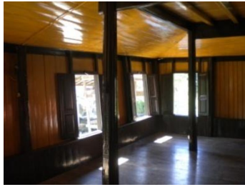
Fig. 3. room in floor I Surau Lubuk Bauk Sources: Personal Documentation.
