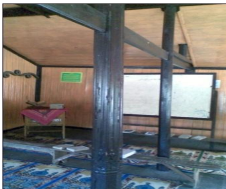
Fig. 7. Wood jeriau that serves to lock the main pillars Sources: Personal Documentation.
