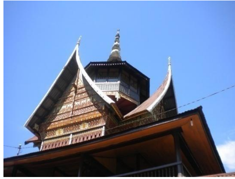
Fig. 8. floor three of surau Lubuk Bauk in form of porch and imbues characteristic of Minangkabau philosophy. Sources: Personal Documentation.
