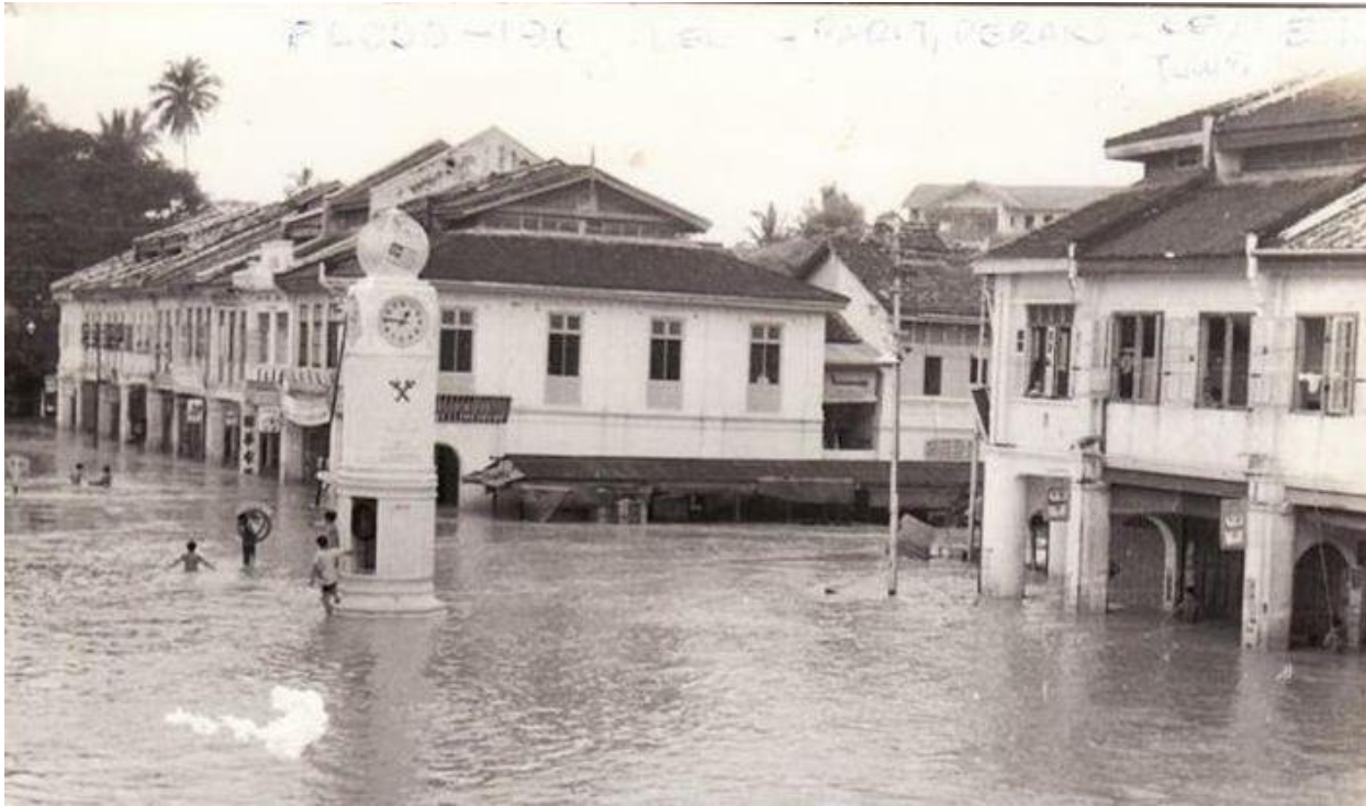
Photo 13: Flooding that occurred in December 1967 Source: www.facebook.com/orgparit
