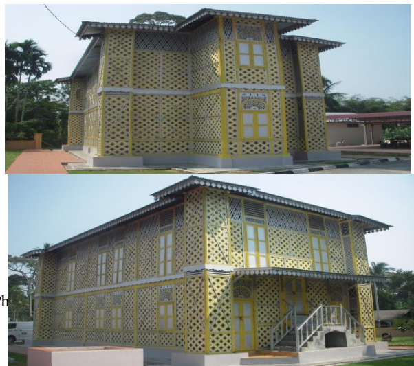
Photo 4.0: The rear elevation of the Kampung Dal Mosque after conservation work Source: Field Work (2012)
