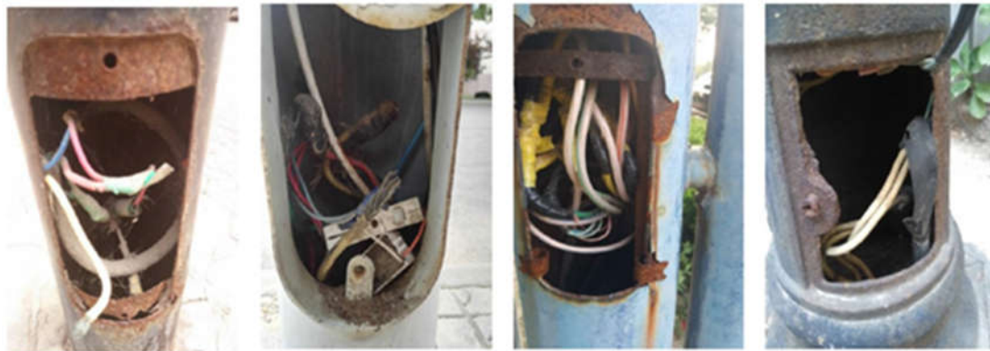
Figure 2: Improper installation of wire in conventional streetlight (Himin Solar Co., Ltd, 2017)
