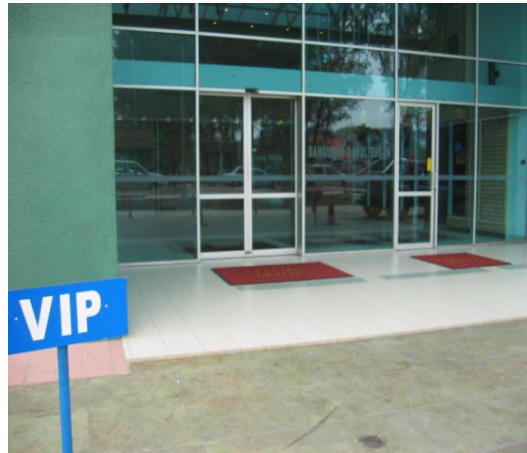
Figure 8: Front Pathways at Darul Ehsan building in Shah Alam
