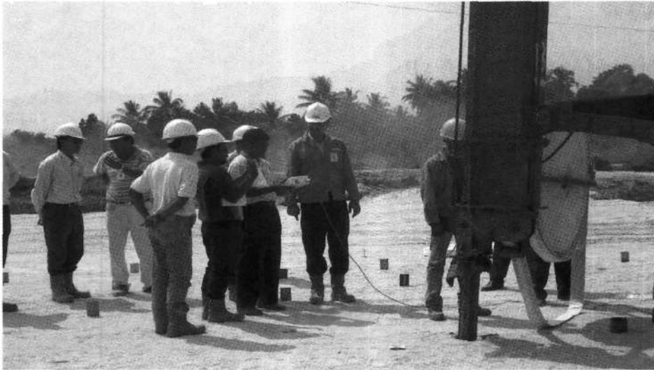
Photo 3 - PVD installation in progress
