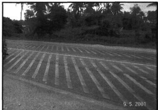
Photo 3: After Installation of Transverse Bar
