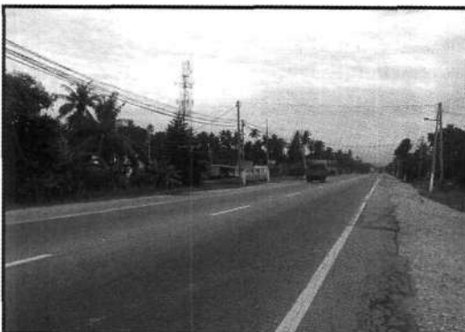
Photo 2: Before Installation of Transverse Bar
