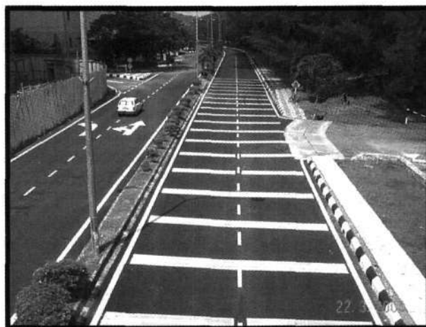
Photo 1: Transverse Bar at Jalan Bangsar
