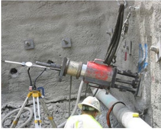
Figure 4: Setup for Pull Out Test
