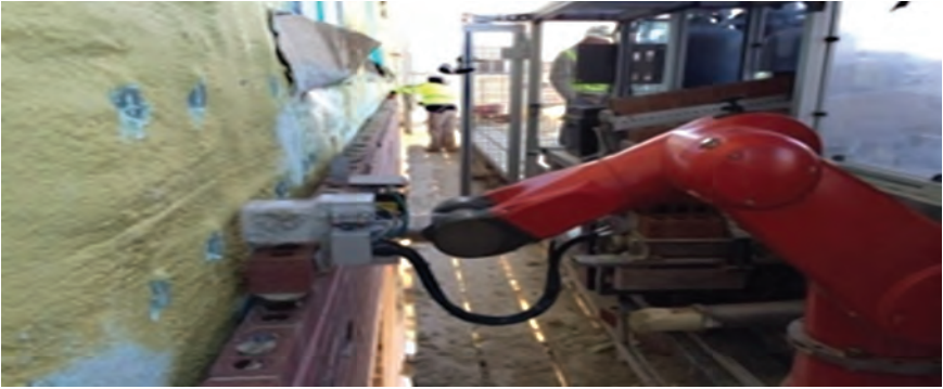
Figure 5: Robotics: Semi-Automated Mason (SAM) is placing a brick (Richard, 2005)
