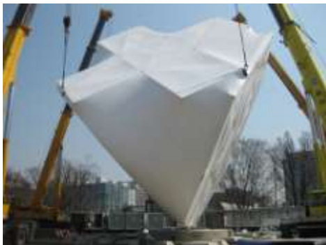
Figure 4: : Exterior structure of Prada Transformer (Futagawa, 2012)
