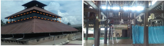
Figure 10: The Roof Aperture Sealed With Plastic and the Fans Installed and Attached to the Wooden Beams
