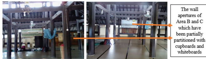
Figure 12: Wall Apertures Partitioned with Cupboards and Whiteboards
