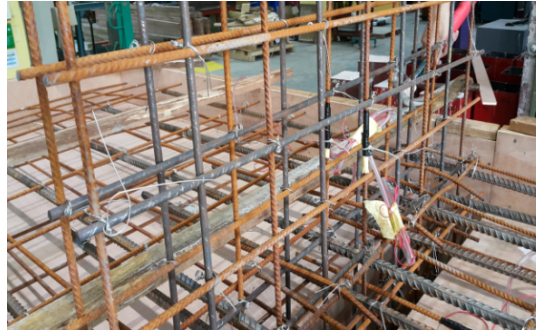
Figure 8: Reinforcement detail of Interior Wall-slab joint
