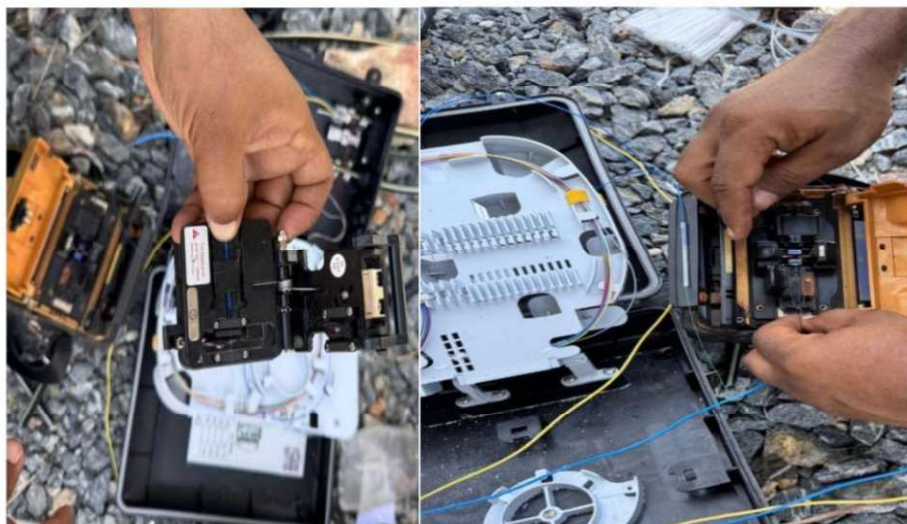
Figure 2: Fiber Optic Preparation and The Fusion Splicing Process
