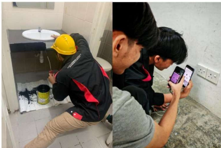
Figure 3: Collaborating With Teammates on Facility Maintenance (Left) and Conducting Safety Inspections of Electrical Outlets (Right)
