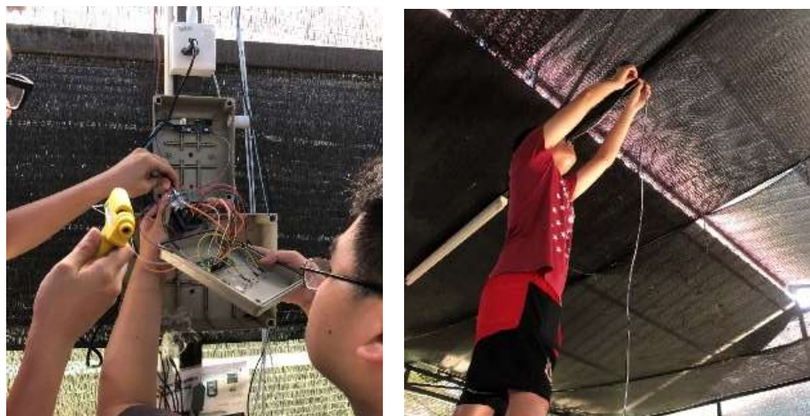
Figure 7. (a) Installation of The Arduino Cover Box (left) and (b) Installation of The DHT22 (right).
