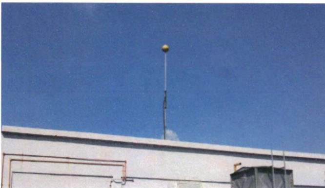
Figure 4: Chancellery UiTM, LPS view (ESE)
