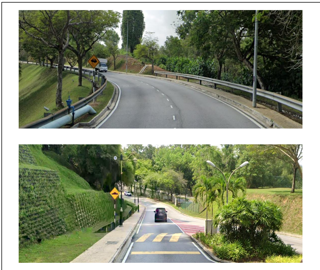
Figure 4.1 Examples of Roadside Hazards, Such as Poles, Trees, and Roadside Distance Severity
