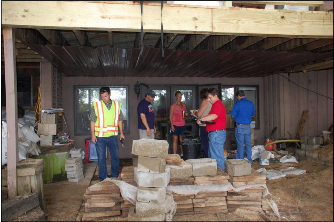
Figure 2.1 Preliminary Damage Assessment (PDA) Team Evaluates Flood Impact near Delhi Dam Failure, Iowa (July 28, 2010)
