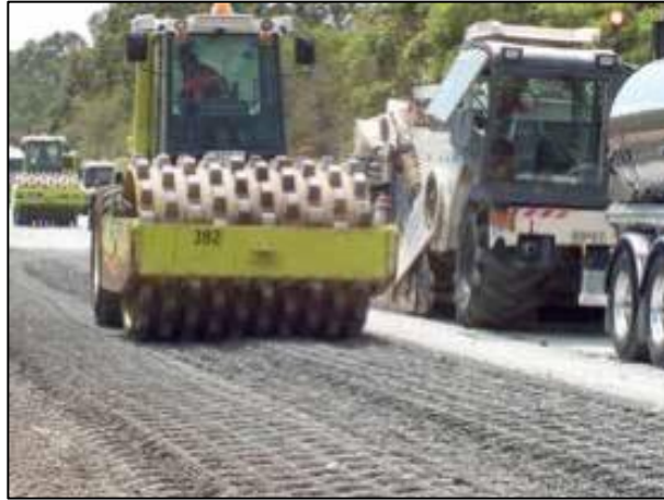
Figure 3-14 The Pad Foot Vibratory Roller
