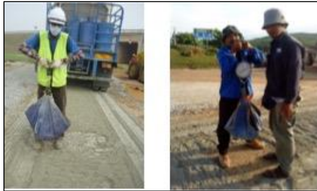
Figure 3-6 Mats/Trays Test on Road (Source: Stabilised Pavements (M) Sdn. Bhd)
