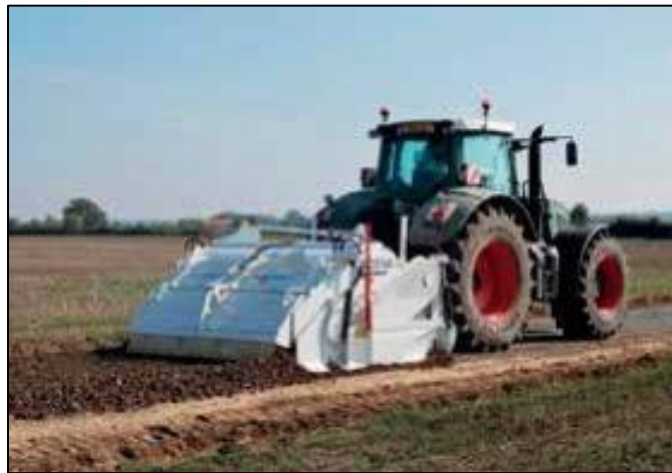
Figure 3-11 Rear-Mounted Mixing Chambers Often Elevate When Encountering Segments of More Rigid Paving Material. (Source: Stabilised Pavements (M) Sdn. Bhd.)
