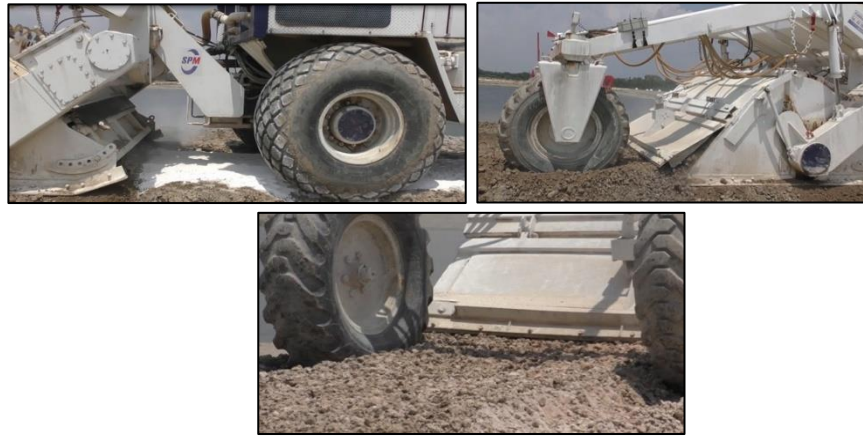
Figure 3-23 In-situ Stabilisation of Marine Clay with 4% Lime (Source: Stabilised Pavements (M) Sdn Bhd.)
