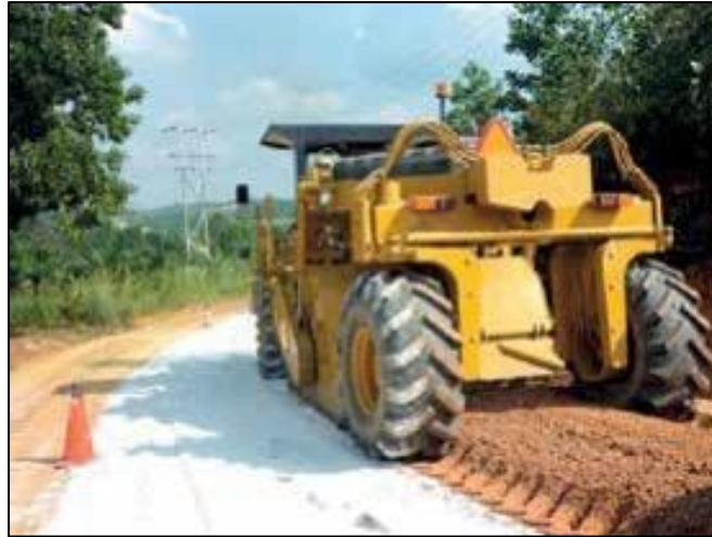
Figure 3-8 After Spreading, The Front Wheels of The Stabiliser or The Rear Wheels of a Centre Drop Spreader Can Move the Binder Sideways (Source: Stabilised Pavements (M) Sdn. Bhd.)
