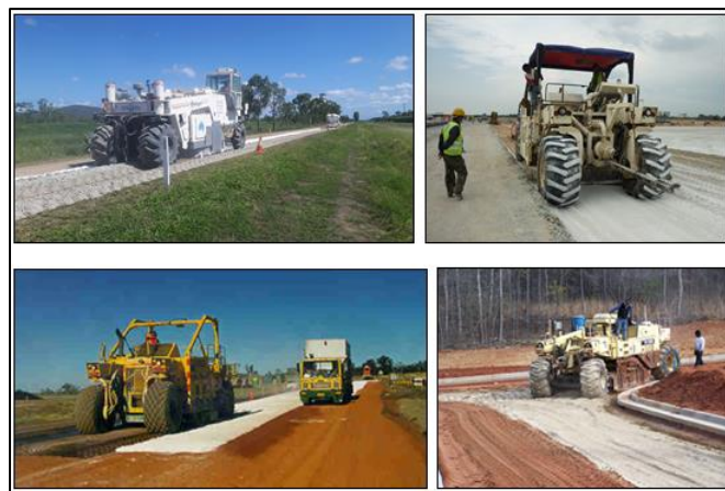
Figure 3-3 Mixing Process for Subgrade Stabilisation Projects
