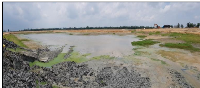
Figure 3-19 Landfill Site (Cell 1) to be Stabilised
