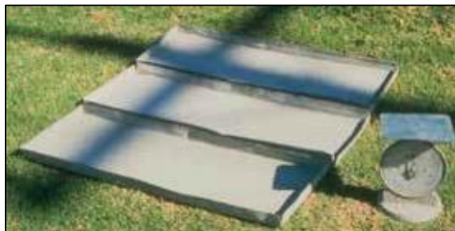
Figure 3-7 Weigh Trays or Mats to Verify the Binder Application Rate
