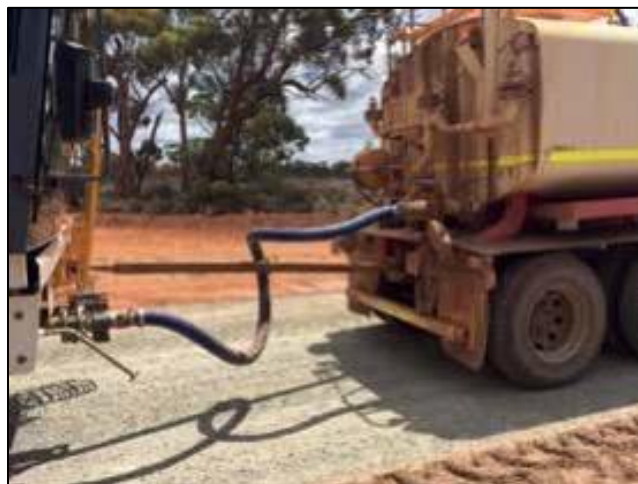
Figure 3-9 The Hose from Tankers to the Stabiliser Will Need to Be Kept from Dragging Using Supports and Chains (Source: Stabilised Pavements (M) Sdn. Bhd.)
