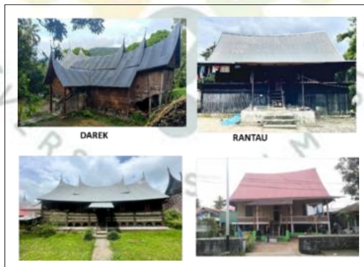
Figure 3: The roof form of darek and rantau
