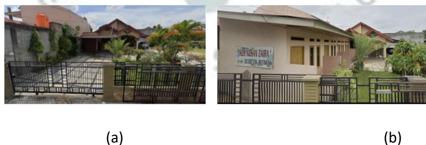
Figure 4: (a) Residential house before expansion, 2022; (b) House with added rental units, 2025. Image Copyright, Google Maps and Author's Survey, 2025
