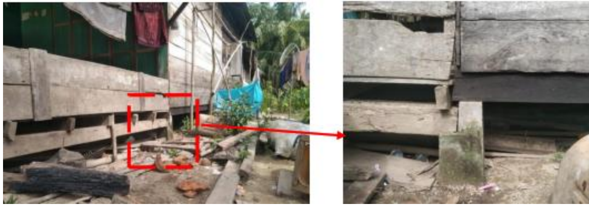
Figure 7: Sandi (Umpak) Foundations in Vernacular Houses in the 1990s.
