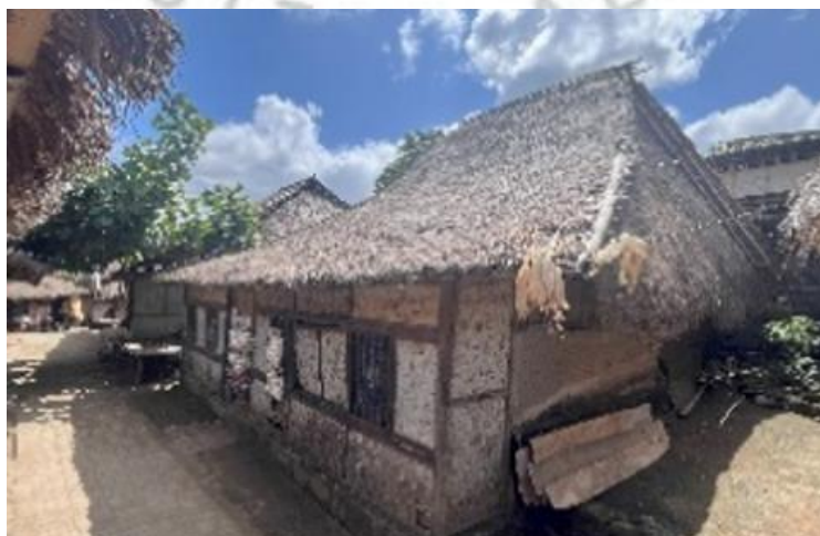
Figure 3: The thatched roof of Bale Tani's house (2025)
