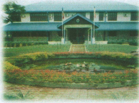
Figure 0.1: the opposite view of the administration building of Agriculture Research Station Tenom
