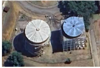
Figure 3 Water Tank UiTM Perak, Branch Seri Iskandar
