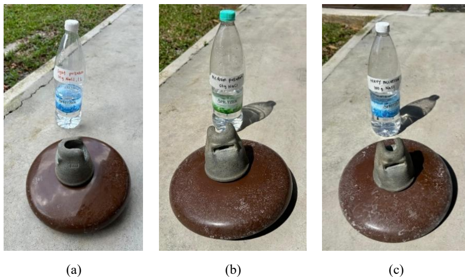
Figure 6. Pollution severity (a) light (b) medium (c) heavy
